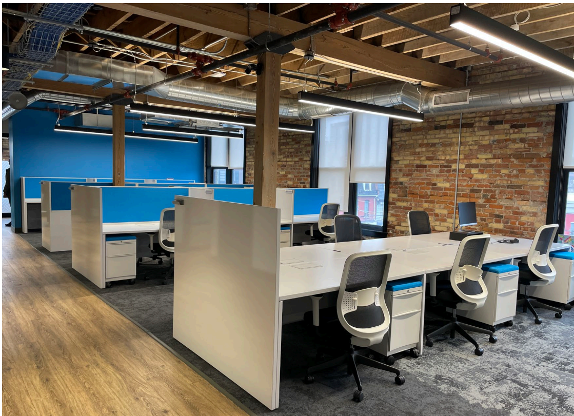
Figure 4. View of the third floor of 339 Queen Street East with beam timber frame construction (Heritage Planning, 2026).
