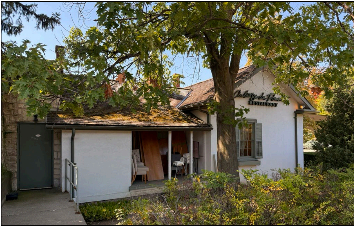
Figure 12. East facade of the former 26 John Street, seen from Yonge Street (Alex Corey, September 2025).
