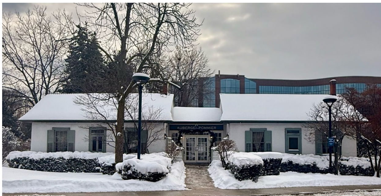
Figure 3. 4150 Yonge Street, north façade (Alex Corey, January 2026).
