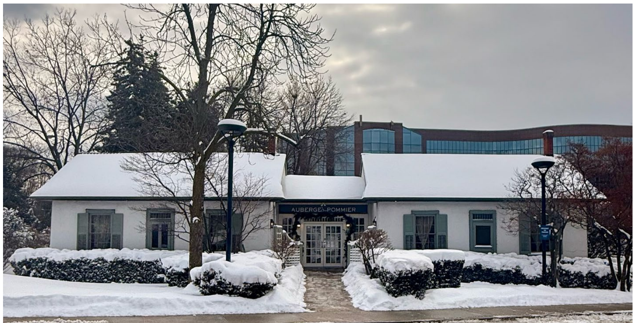
Figure 2. 4150 Yonge Street, north façade (Alex Corey, January 2026).
