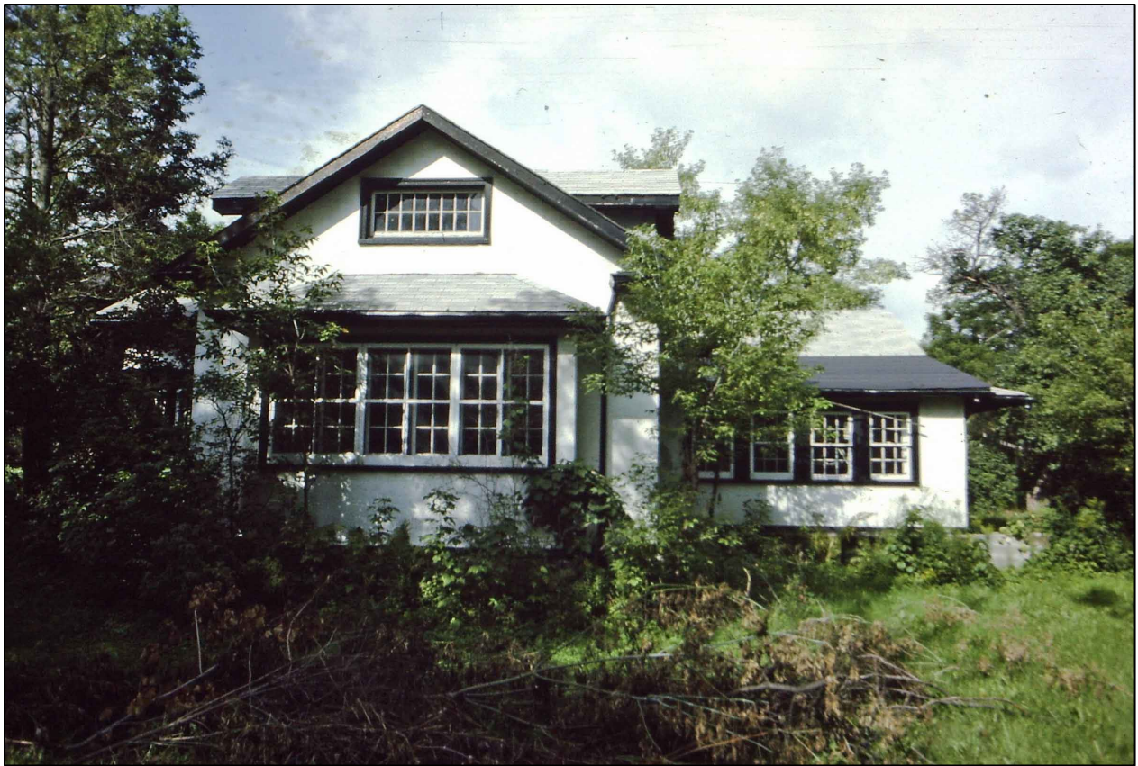
Figure 6. 22 John Street, east facade, 1977. Toronto Historical Board.
