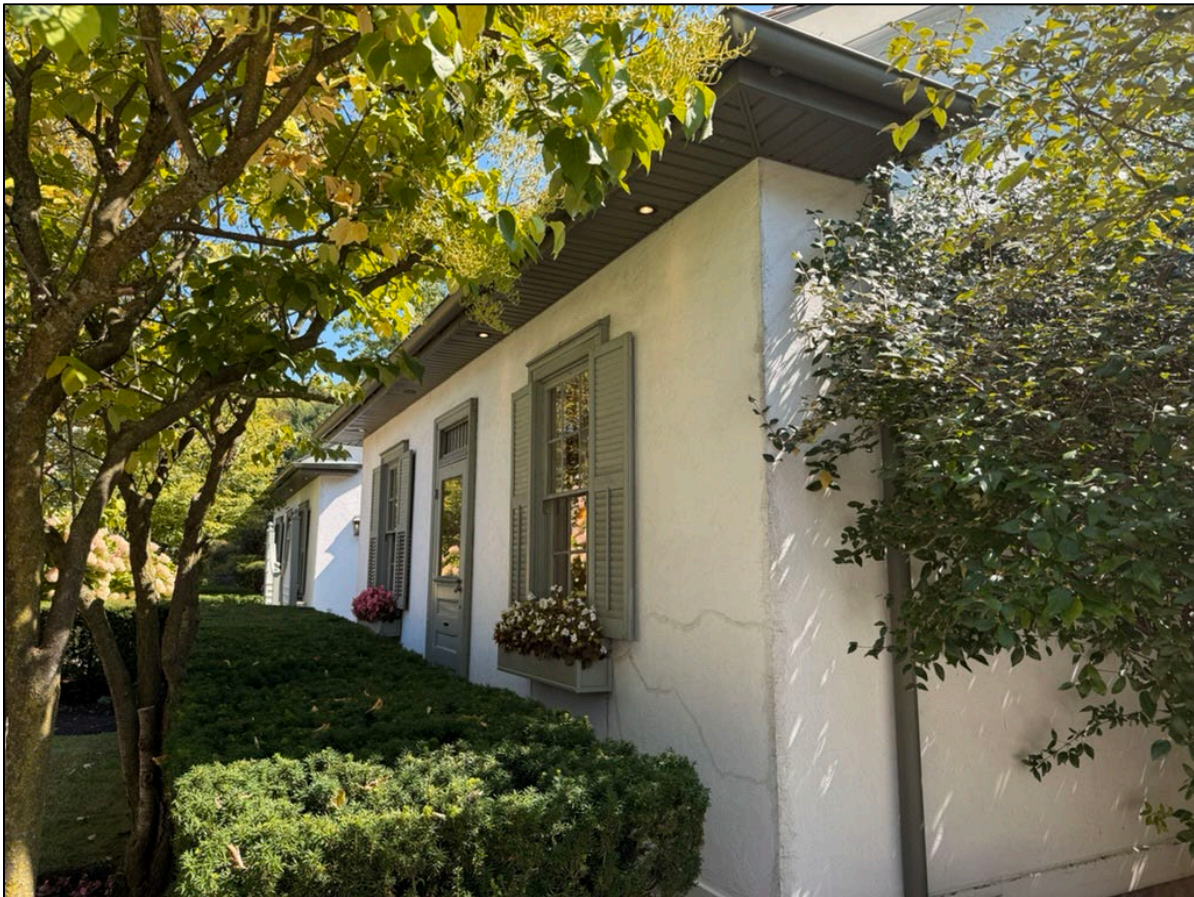
Figure 13. Primary (north) facade of the former 22 John Street (Alex Corey, September 2025).
