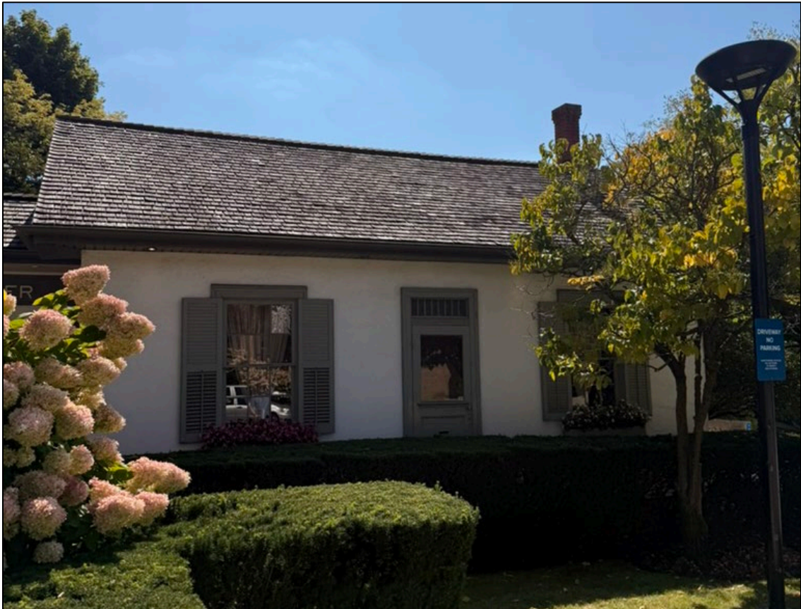
Figure 11. Workers Cottage formerly at 22 John Street, now the western cottage of the two (Alex Corey, September 2025).
