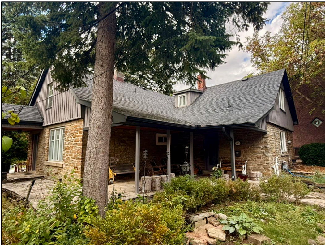
Figure 2. 34 Jason Road, southeast façade (Alex Corey, September 2025).
