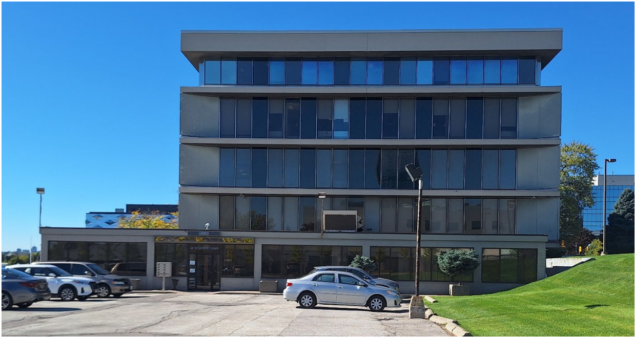
Figure 12 East elevation of 39 Wynford Drive with basement addition. Note the southward sloping landscape (Heritage Planning, 2025).
