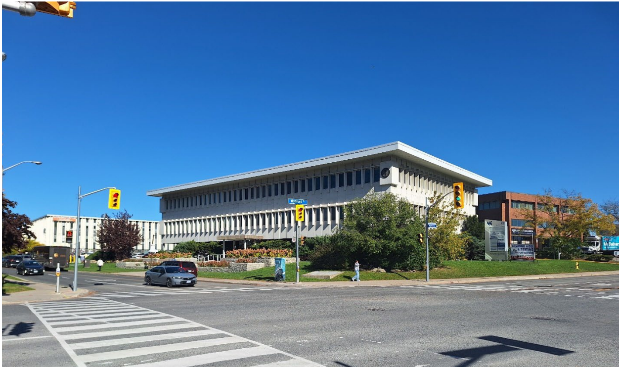
Figure 15 View looking northeast from the intersection of Wynford Drive and Gervais Drive towards 20 Wynford Drive (Heritage Planning, 2025).
