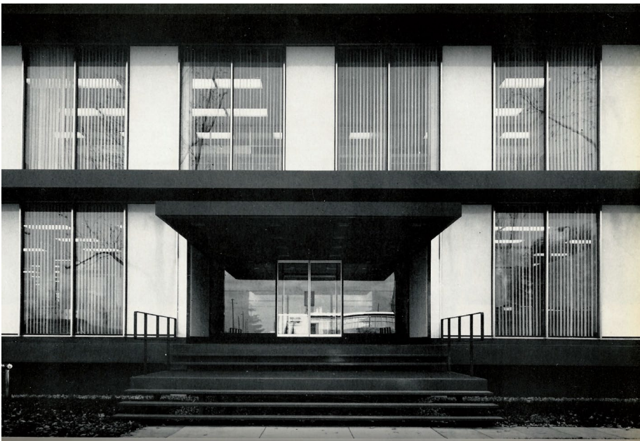
Figure 3(a) 1960s image showing the main entrance (The Canadian Architect 1963:60)
