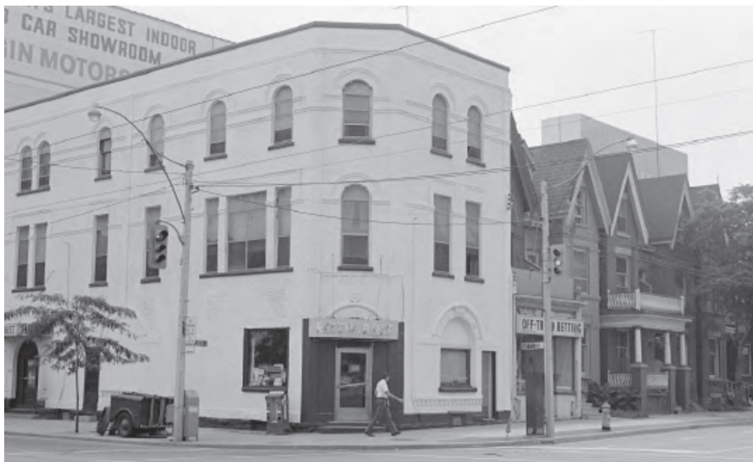
Figure 8: 1972 archival photograph, looking southwest from Bay and Elm streets at the north and east elevations of the property. (City of Toronto Archives)
