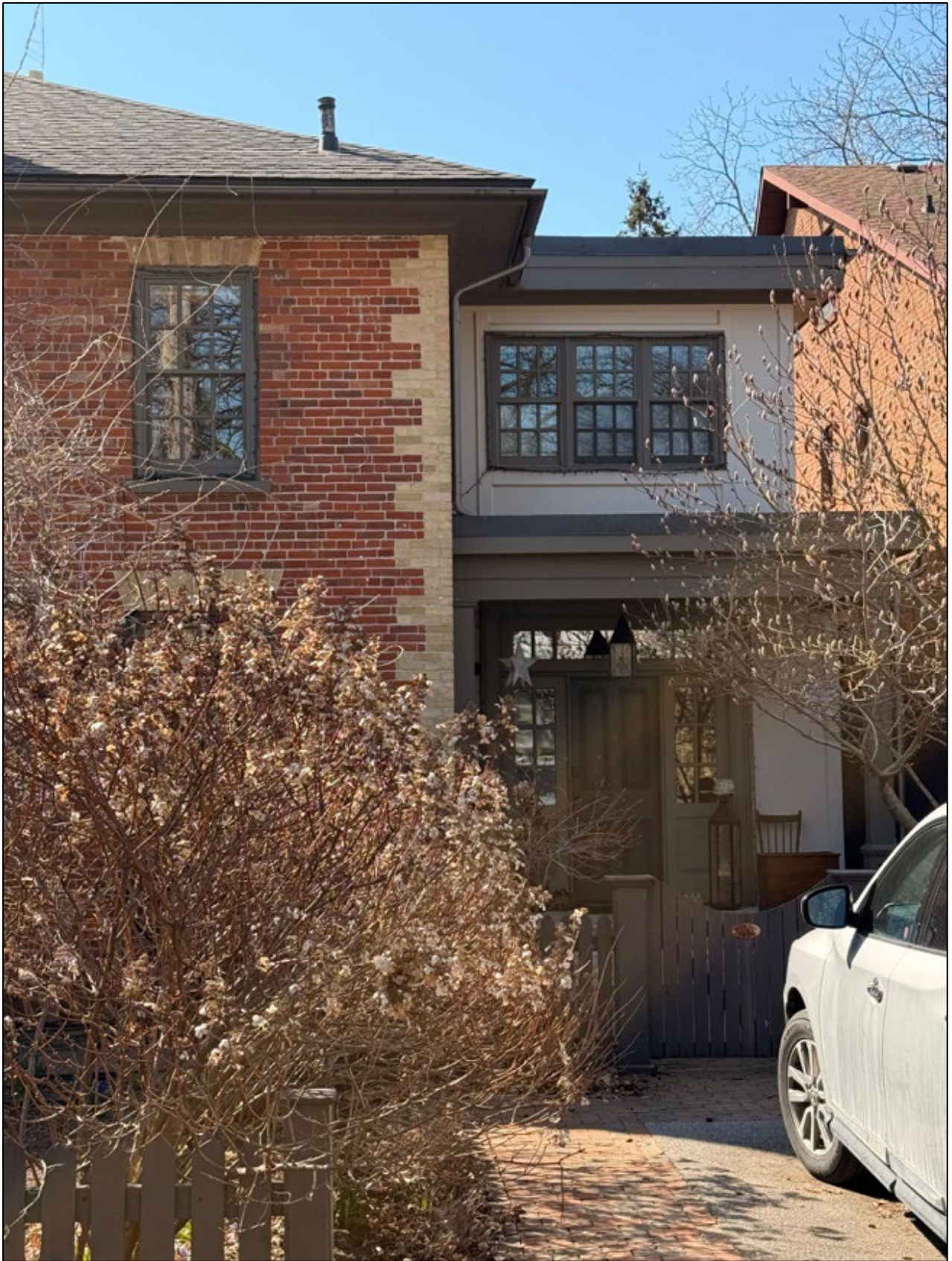
Figure 19. 7 Meadowcrest Road, rear (west) 2-storey addition (Alex Corey, April 2026).
