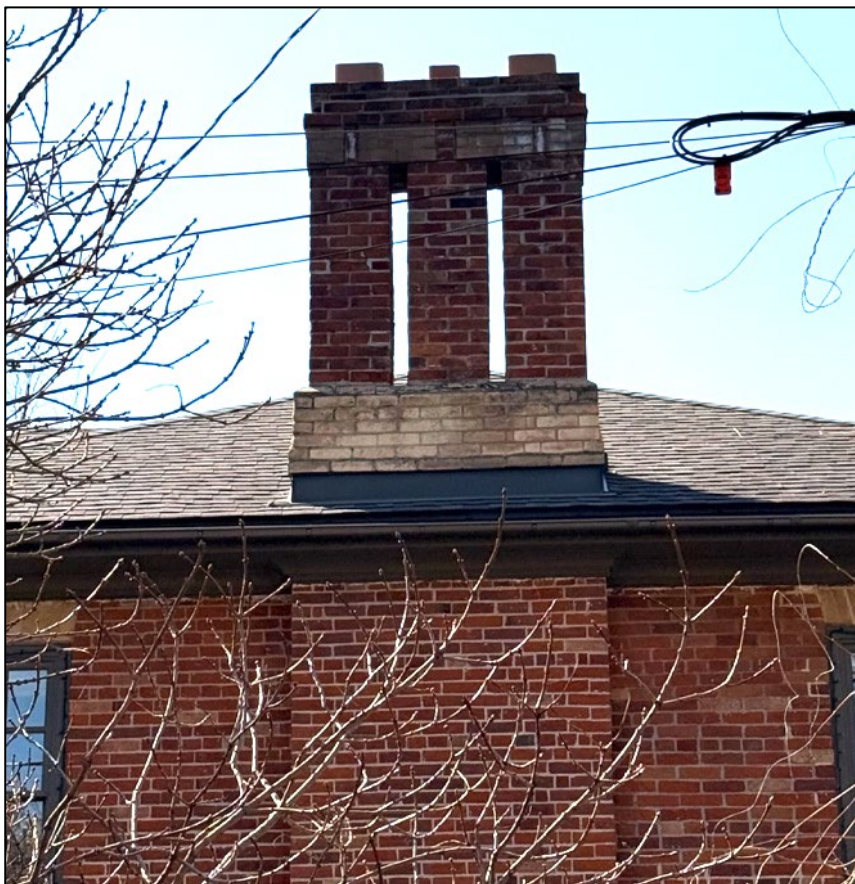
Figure 17. 7 Meadowcrest Road, north chimney with polychrome brick detailing (Alex Corey, April 2026).
