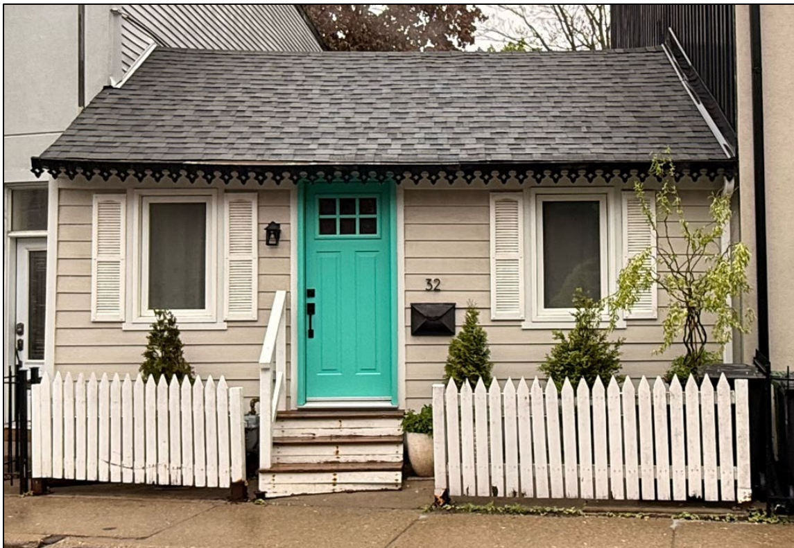
Figure 3. 32 Bright Street, primary (east) elevation (Alex Corey, May 2026).
