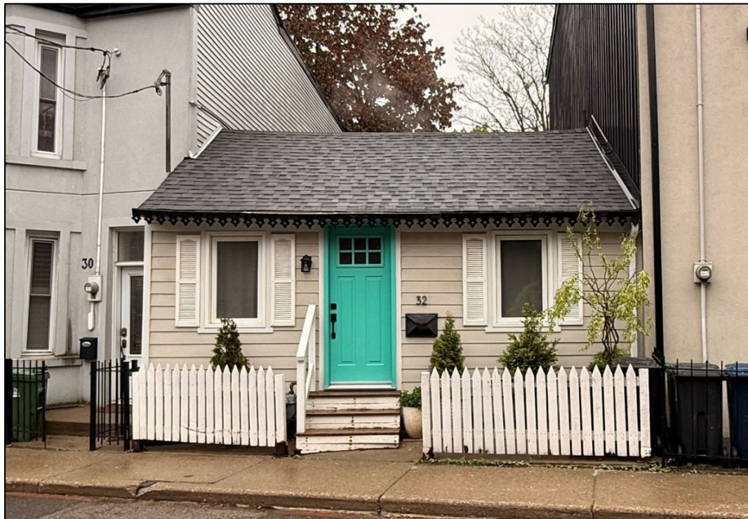
Figure 2. 32 Bright Street, primary (east) elevation (Alex Corey, May 2026).
