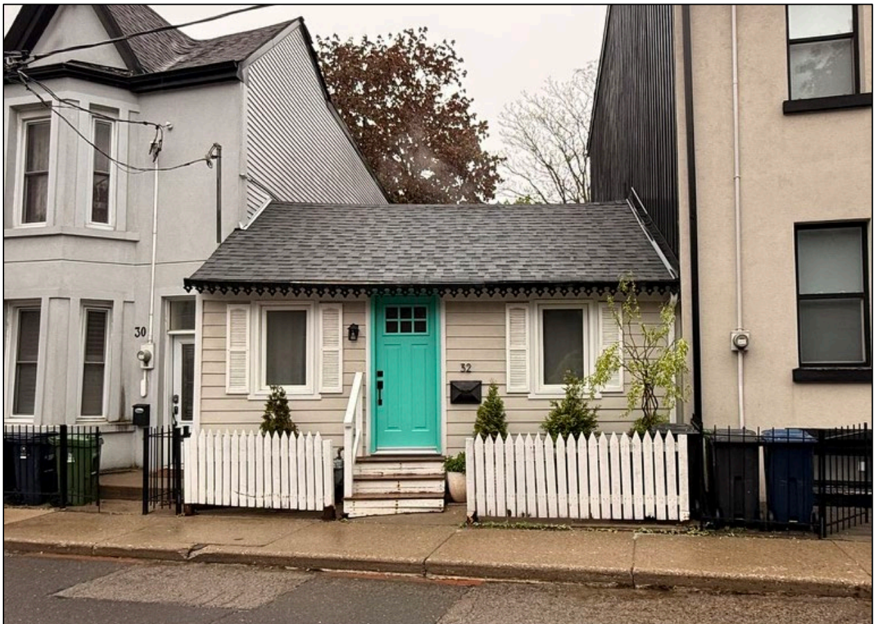
Figure 16. 32 Bright Street, primary (east) elevation (Alex Corey, May 2026).
