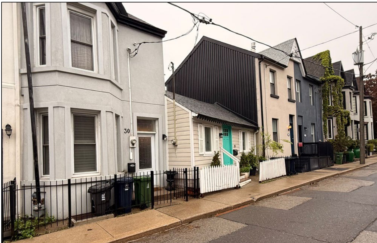
Figure 18. View looking northwest towards 32 Bright Street, showing the rowhouses immediately to the north (Alex Corey, May 2026).
