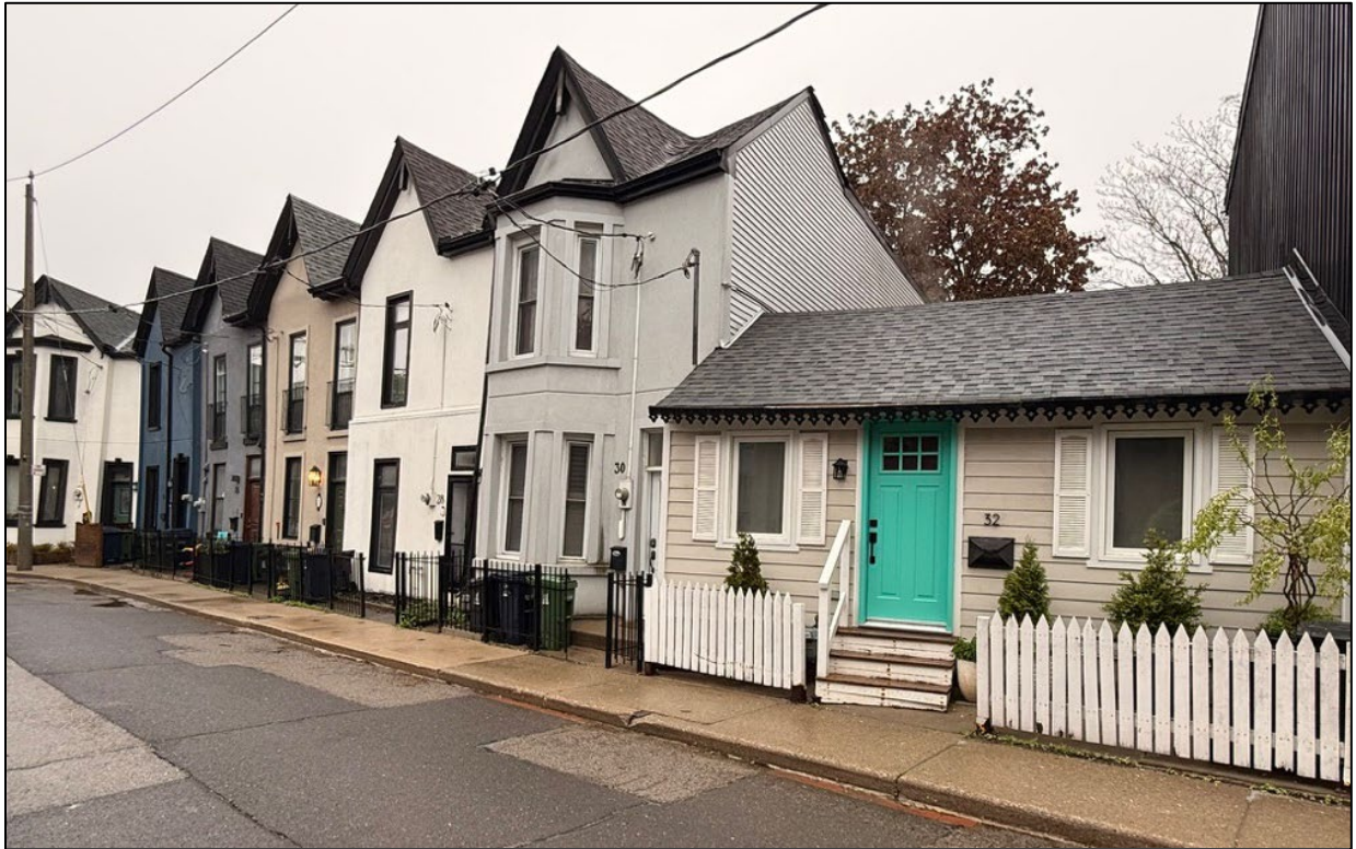
Figure 17. View looking southwest to 32 Bright Street, showing the rowhouses immediately to the south (Alex Corey, May 2026).
