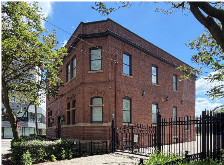
Oblique view from northwest of 55 Sudbury Street, 2026 (City of Toronto Heritage Planning)
