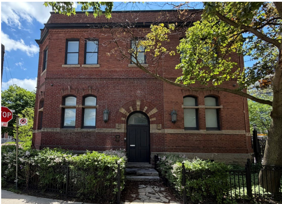
55 Sudbury Street, 2026 (City of Toronto Heritage Planning)
