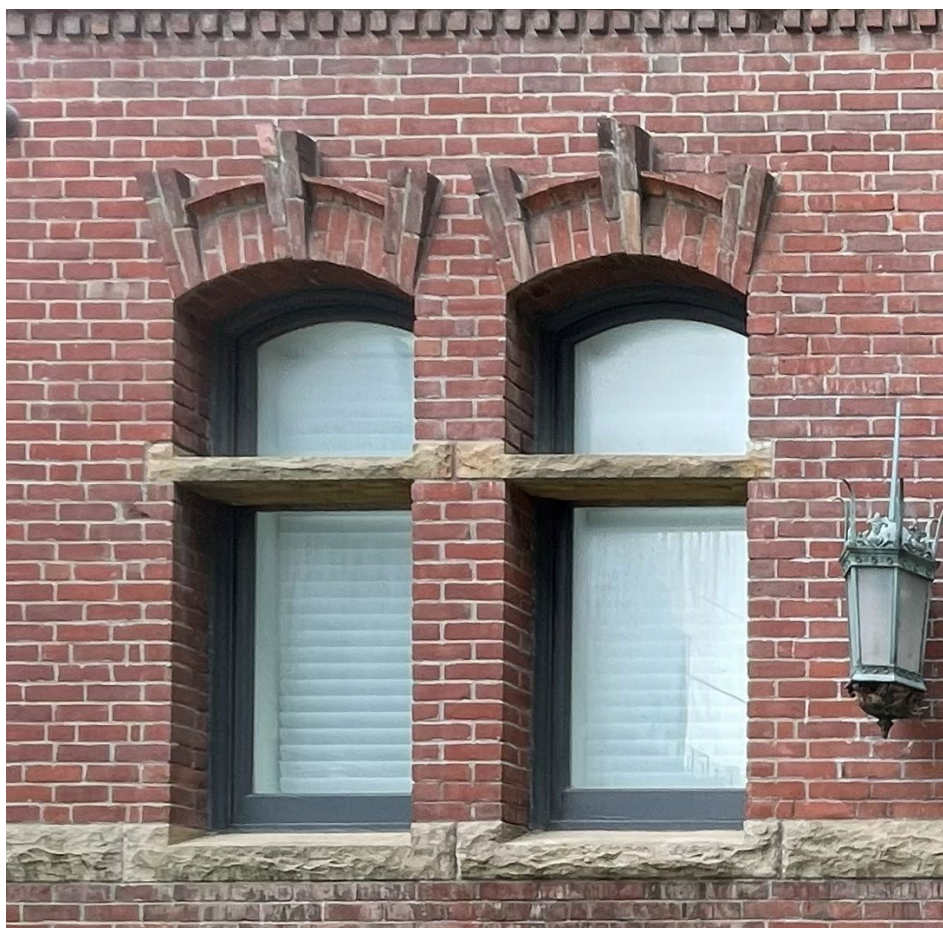
Figure 6: Example of window detailing, north façade, 2026 (City of Toronto Heritage Planning)
