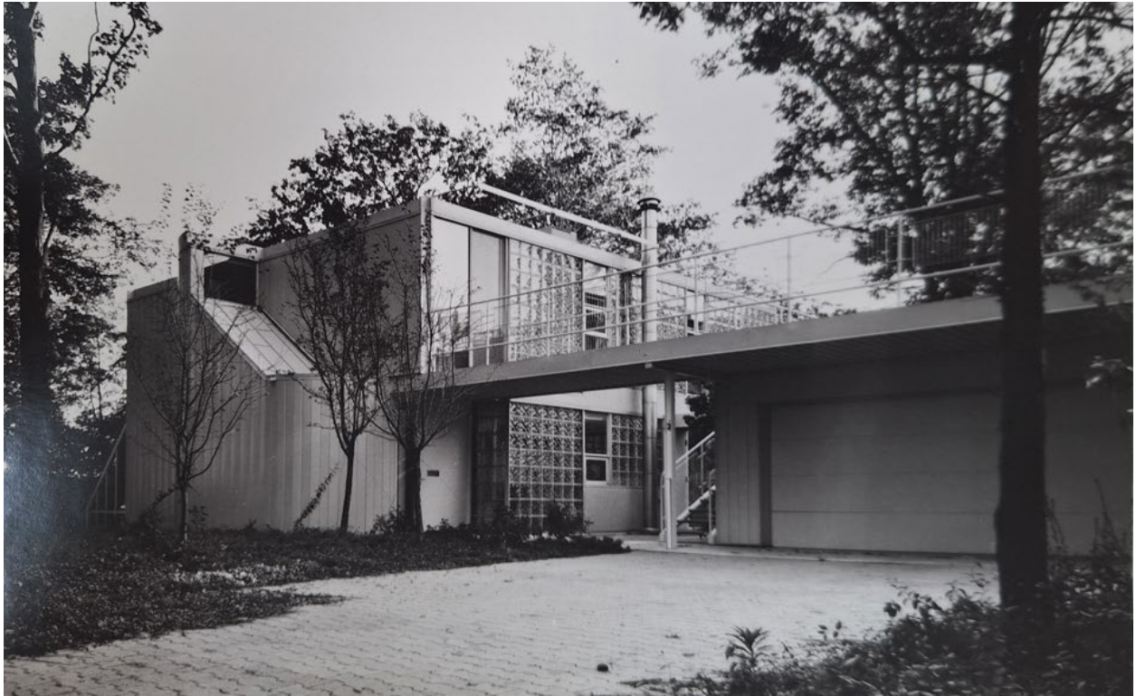
Figure 1 Archival image of the east and north elevations of 2 Hedgewood Road. Note the front verandah extending across the garage and courtyard with pipe railing, glass block walls of the north elevation, and exterior mounted chimney (City of Toronto Archives).
