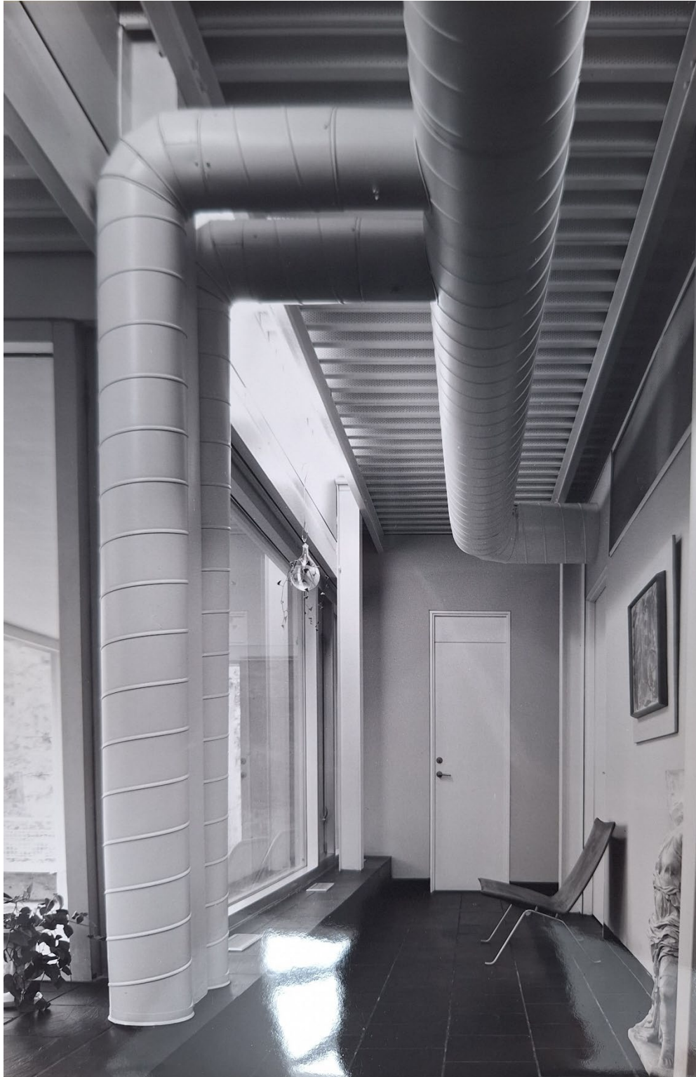
Figure 17 Archival image of basement hallway showing exposed ductwork and exposed steel ceiling (City of Toronto Archives).
