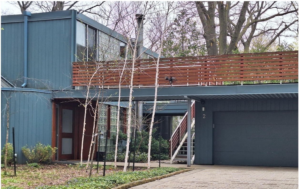
Figure 7 View looking west towards the courtyard. Note the staircase railing has been overclad in wood slats (Heritage Planning, 2026).
