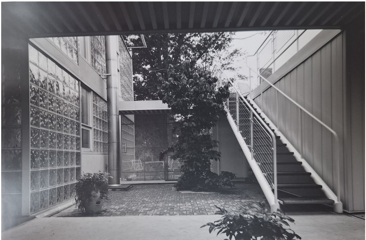
Figure 6 Image looking west from the front verandah showing the central courtyard with exterior staircase, pipe railings, exterior mounted chimney and rear verandah with sliding metal mesh doors (City of Toronto Archives).
