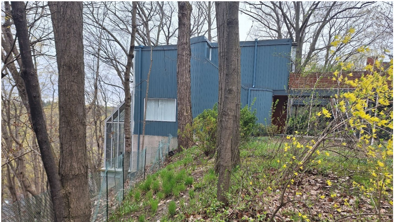
Figure 5 View of the east elevation of the house at 2 Hedgewood Road showing the two-storey bay overlooking the West Don River Valley (Heritage Planning).
