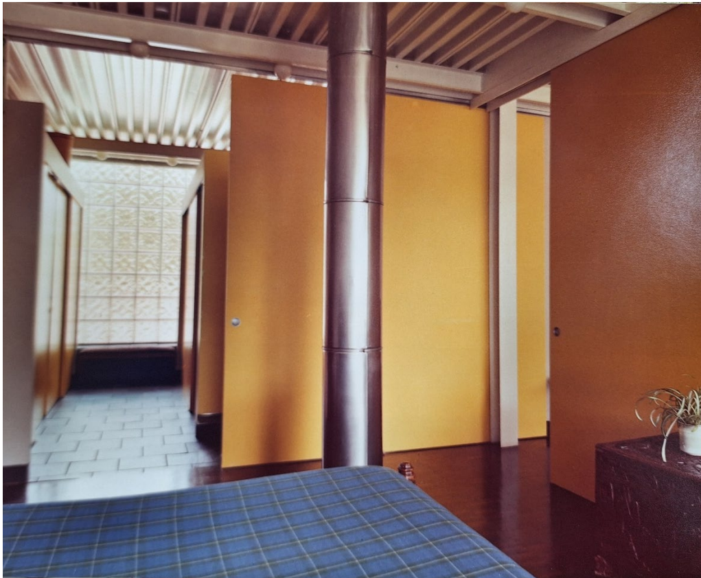
Figure 16 Archival photo of second-storey bedroom with exposed ductwork and steel ceiling and support columns (City of Toronto Archives).
