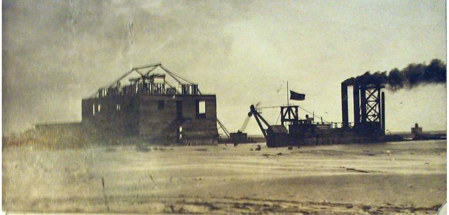
Second NYC clubhouse under construction (1919)
