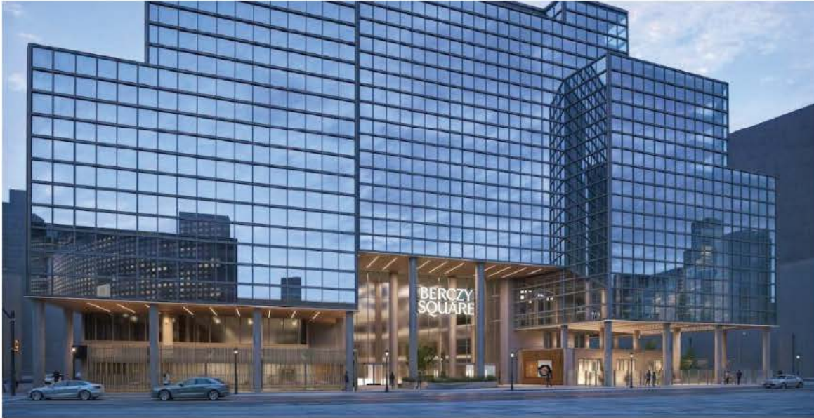
Figure 1: West Elevation of Site
