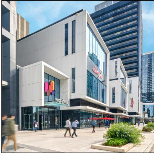
Figure B: Yonge Sheppard Centre N.E. corner.
