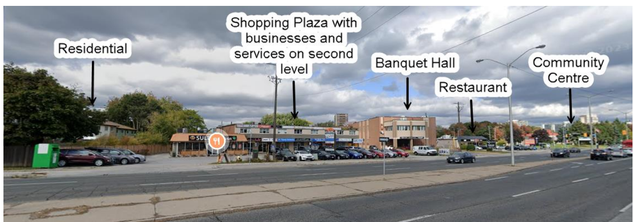
Image #7: A Picture Of The Immediate Adjacent Neighbouring Property Directly East Of The Proposed Premises, Zoned CR Sign District
