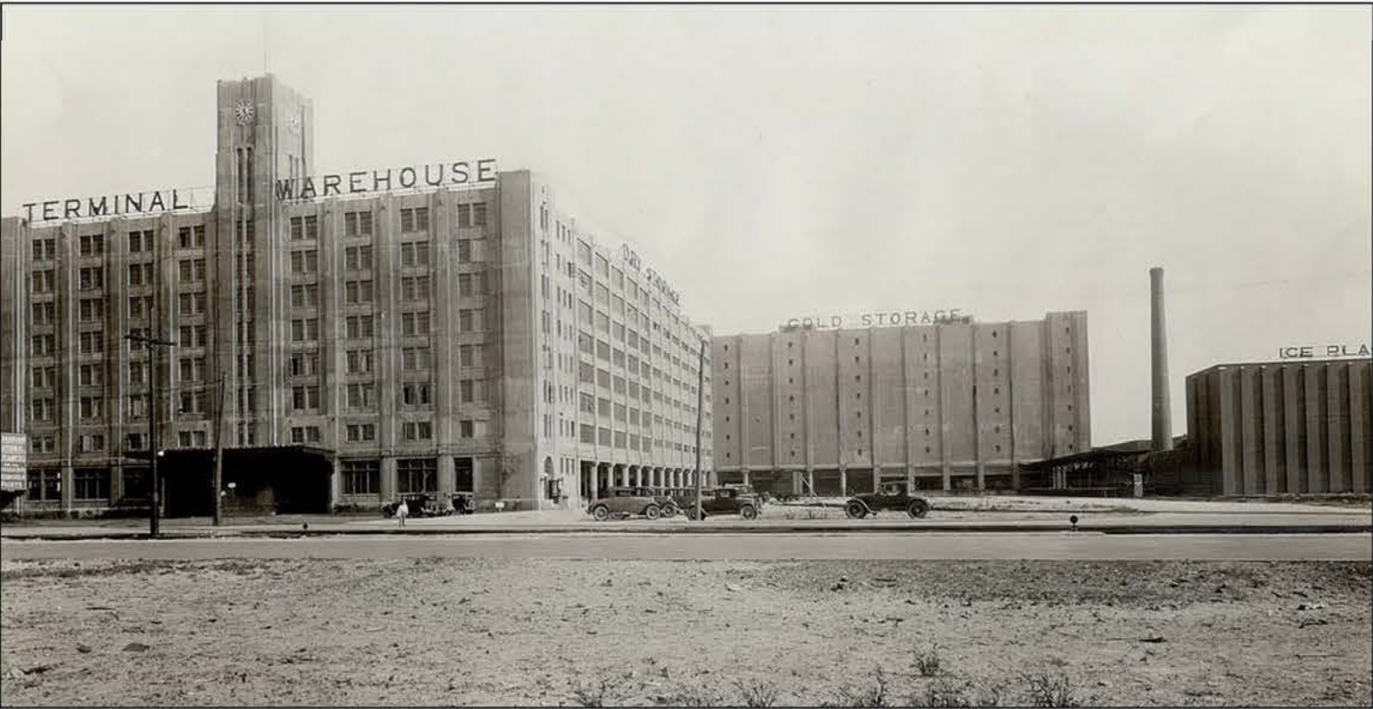
1 Terminal Warehouse Letters W1.0c Date: 1929
