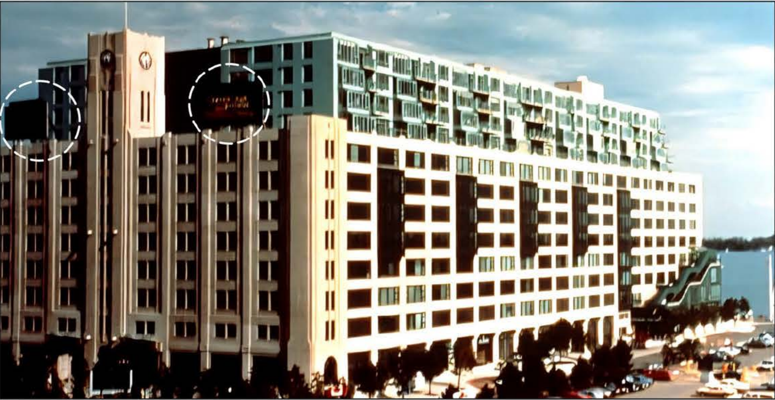
3 Rooftop Billboards W1.0c Date: 1970s
