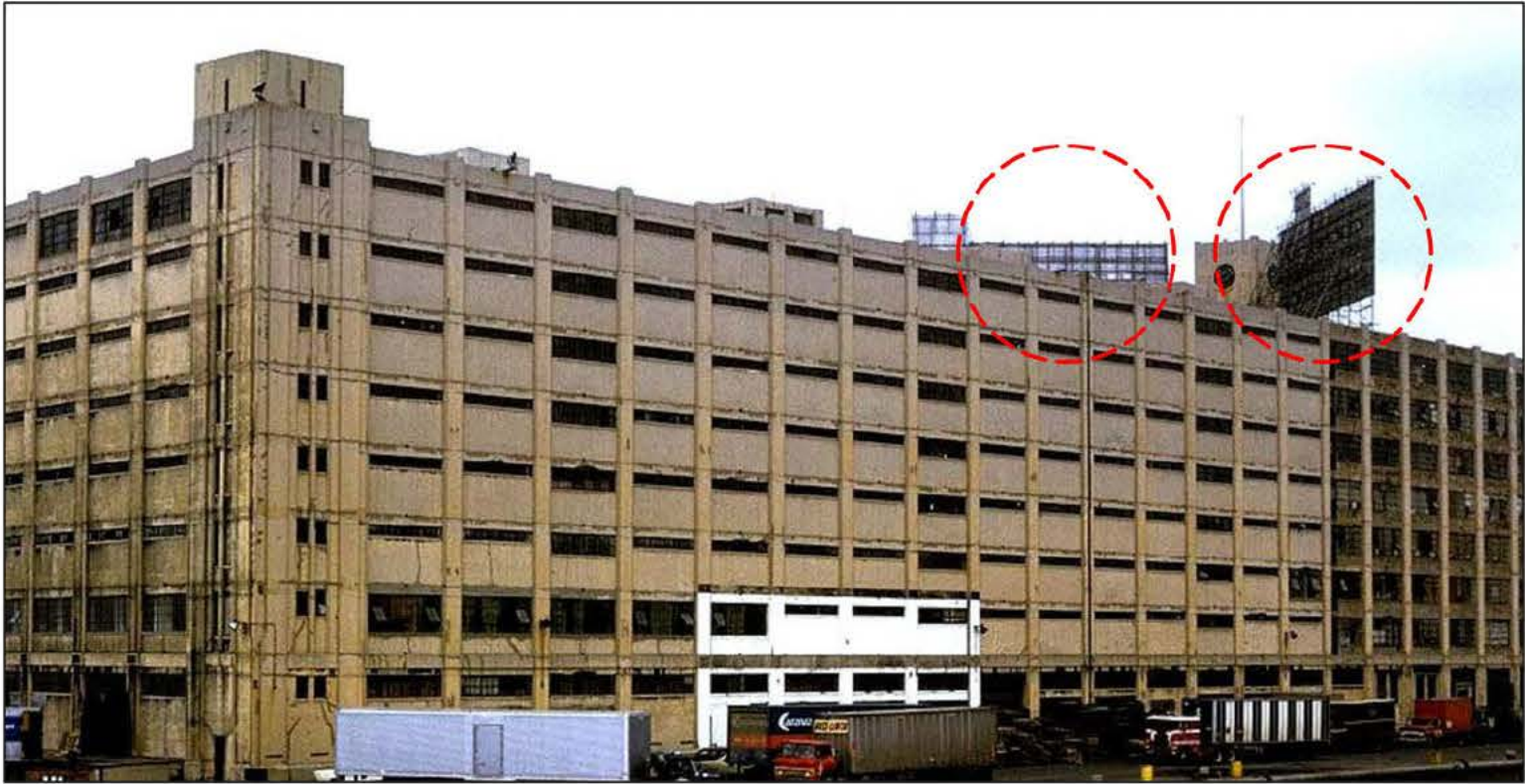
4 Rooftop Billboards W1.0c Date: 1970s
