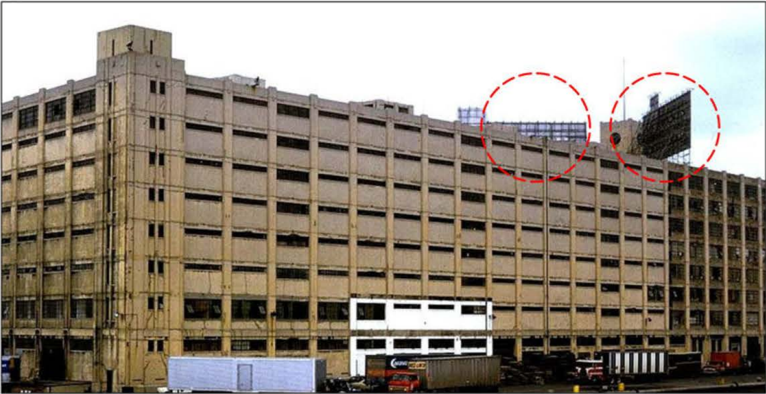
4 Rooftop Billboards W1.0c Date: 1970s
