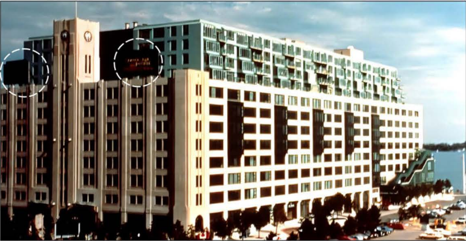
3 Rooftop Billboards W1.0c Date: 1970s
