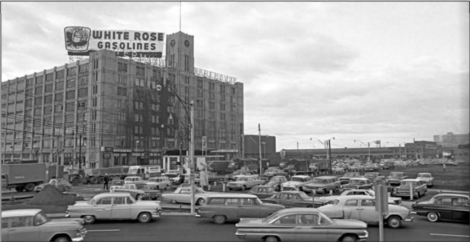
2 Terminal Warehouse Letters and Roof top Billboard W1.0c Date: 1963
