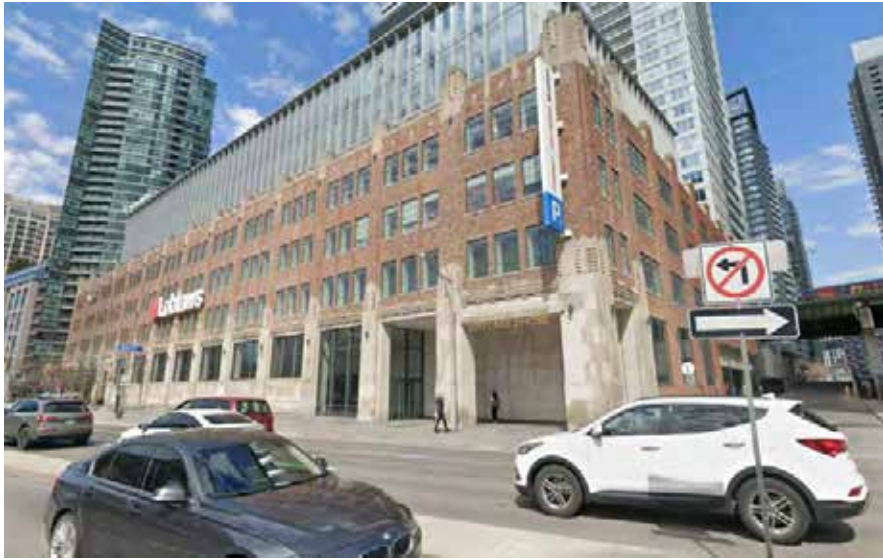
Photo 19. 500 Lake Shore Boulevard West (Loblaws Groceries Company) with projecting sign at southeast corner of building and custom formed box sign on south elevation (Google Maps, 2026)
