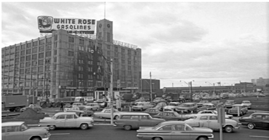
Photo 4. 1963 photograph of Terminal Warehouse with signage for "White Rose Gasolines" at roof level and tall wall mounted sign at west pilaster on north elevation (Google)
