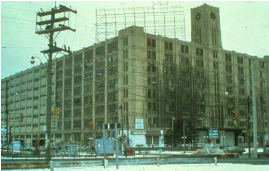
Photo 6. c. 1980s photograph of Terminal Warehouse with unused signage support structure at roof level and wall mounted sign at east pilaster on north elevation (City of Toronto Archives)
