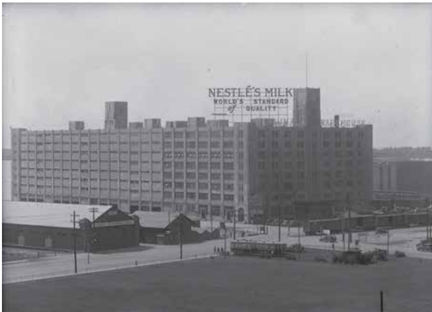
Photo 2. 1930 photograph of Terminal Warehouse with signage for "Nestlé's Milk" at roof level and projecting sign at east pilaster on north elevation (Library and Archives Canada)
