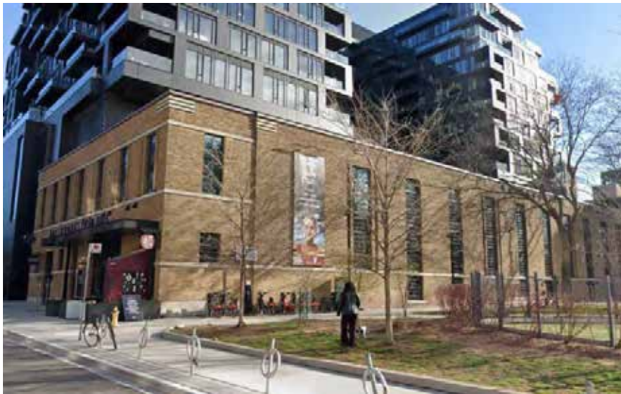
Photo 20. 497 Richmond Street West (Water Works Building) with wall mounted banner sign at west end of south elevation (Google Maps, 2026)
