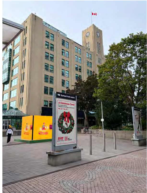
Photo 13. View of the Site looking southwest from Queen's Quay West (ERA, 2026)
