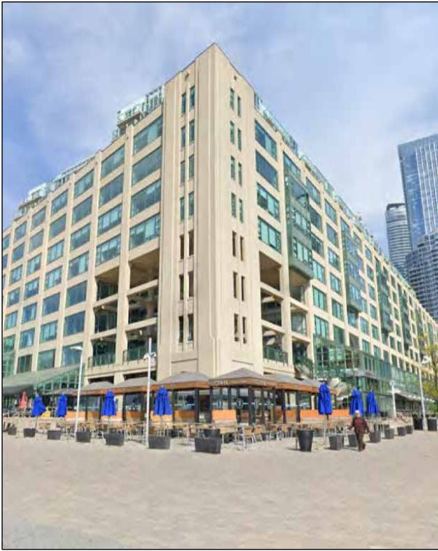
6 Southeast Corner Looking North W1.0f
