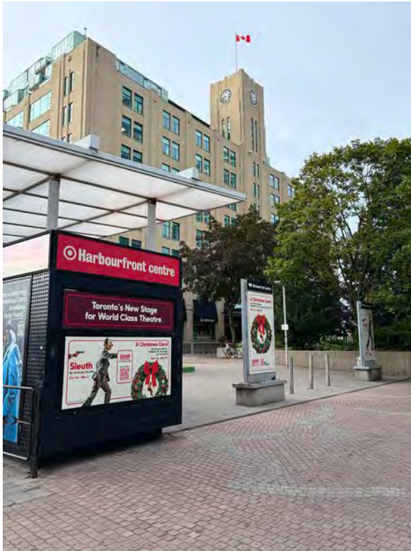
Photo 12. View of the Site looking southwest from Queen's Quay West (ERA, 2026)
