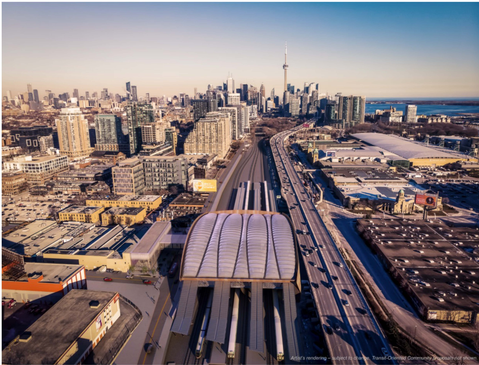
Future Exhibition Station aerial view looking east, featuring shared GO/Ontario Line station building and platforms in foreground.
