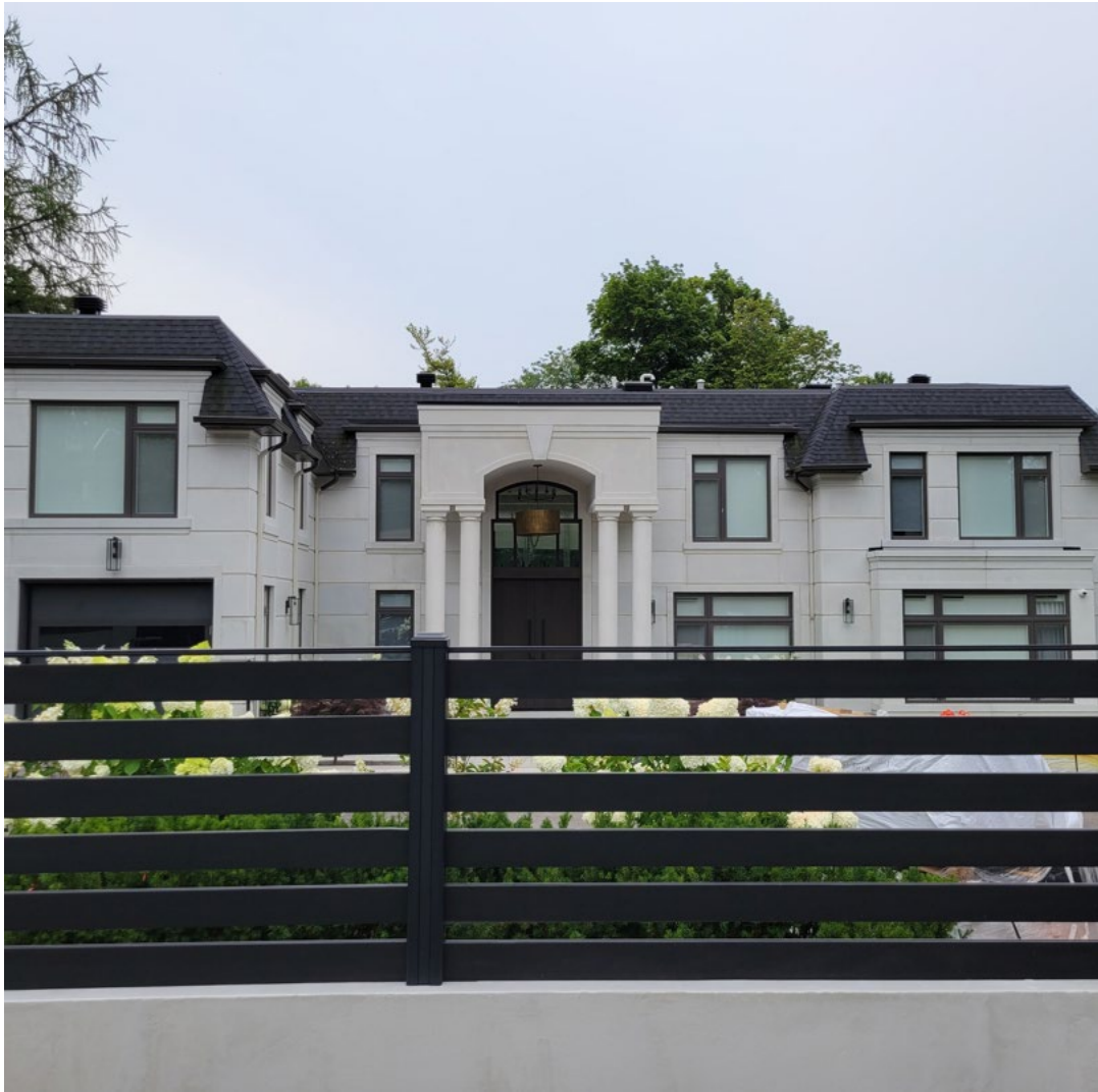
Attachment 7: Fence between Gates
