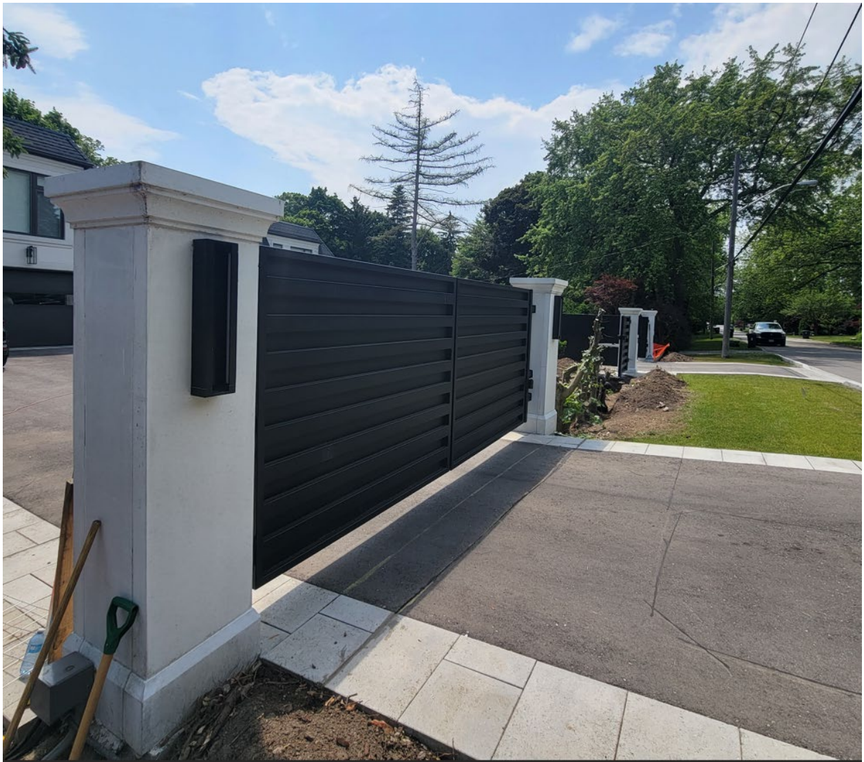
Attachment 2: North Property Line Gates with Pillars
