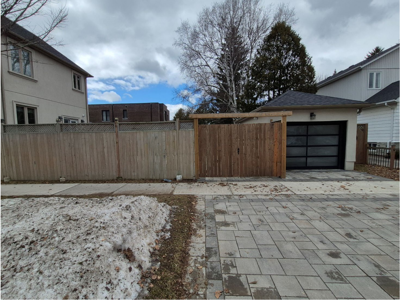
Attachment 2: Supervisor's photo -Overview of fence at 120 Donside Road.
