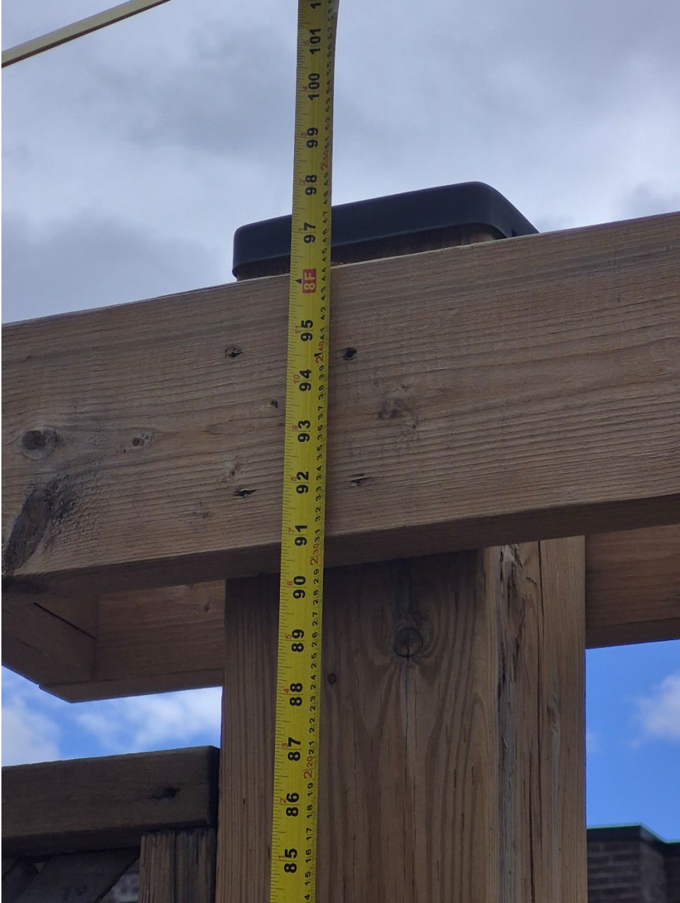
Attachment 4: Supervisor's photo - Fence Height (2.48 meters)
