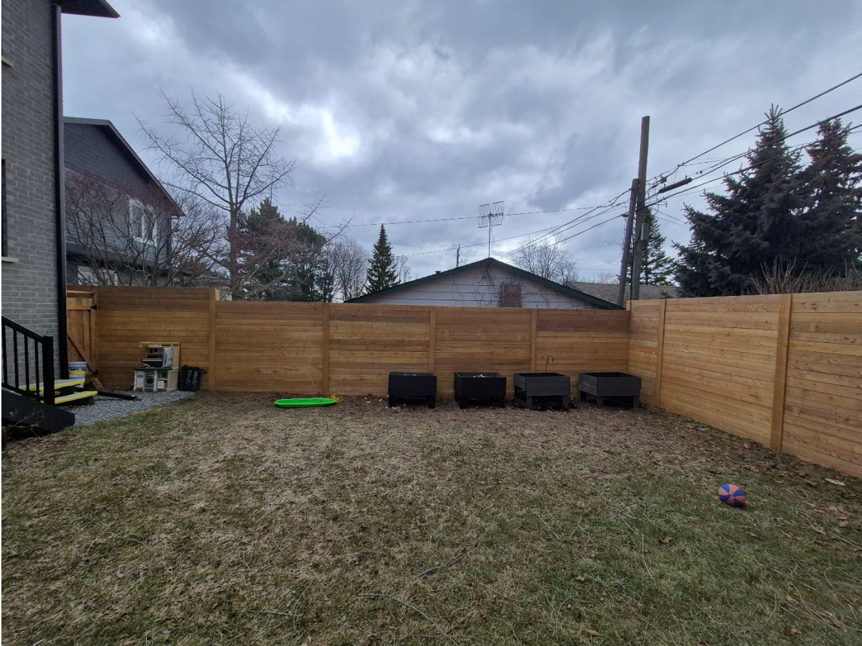
Attachment 9: Supervisor's photo - Overview of south fence at 4 Brooklawn Avenue
