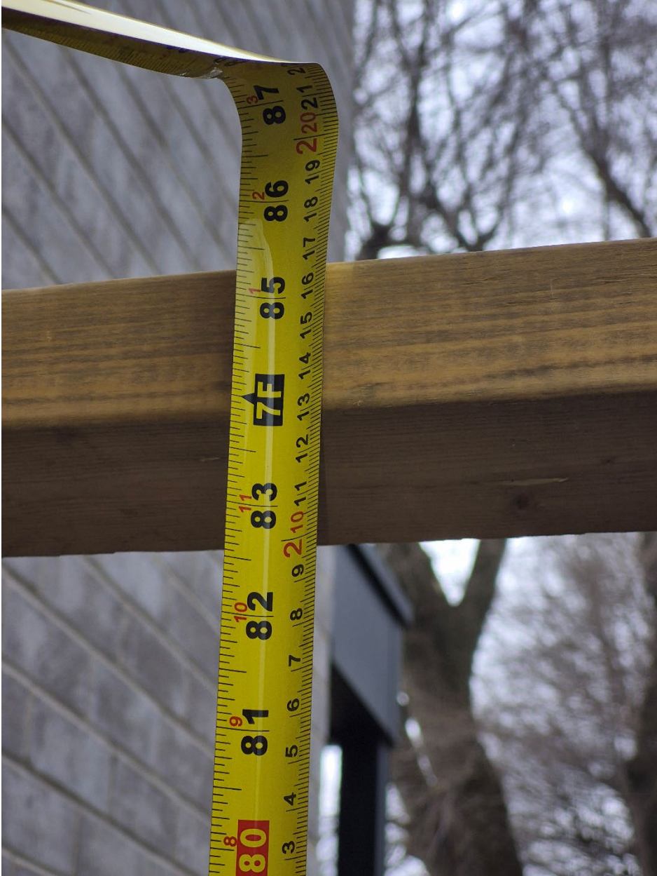
Attachment 3: Supervisor's photo - North gate height (2.17 meters)
