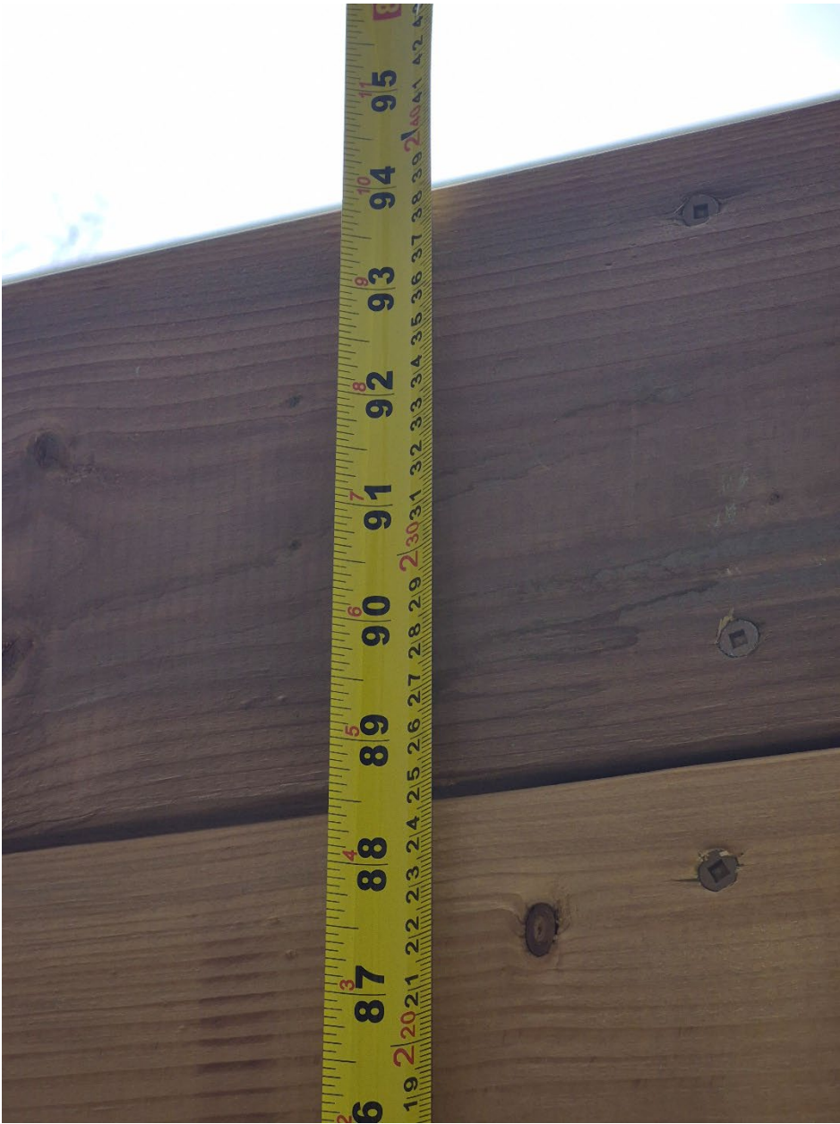
Attachment 6: Supervisor's photo - North fence height (2.39 meters) at 4 Brooklawn Avenue
