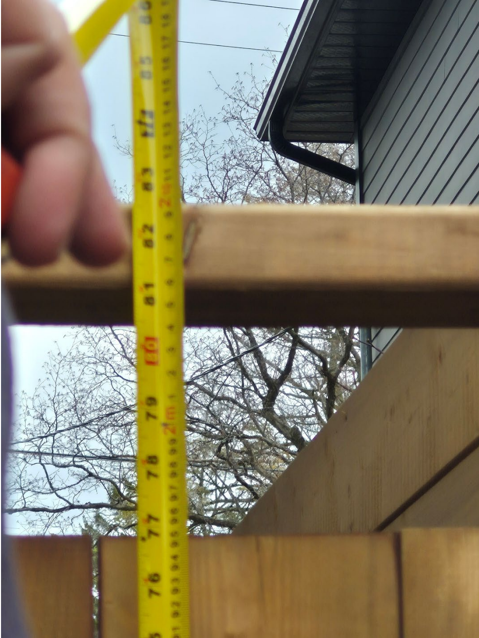
Attachment 12: Supervisor's photo - South gate height (2.1 meters)
