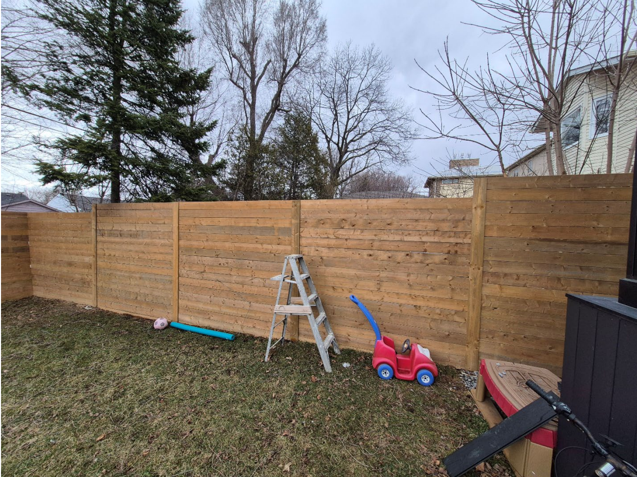
Attachment 5: Supervisor's photo - Overview of north fence at 4 Brooklawn Avenue
