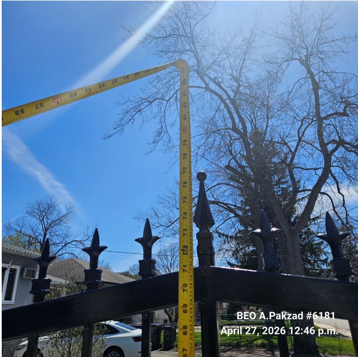
Attachment 6: Supervisor Photo – Height of South Fence (Close up) (1.95m)
