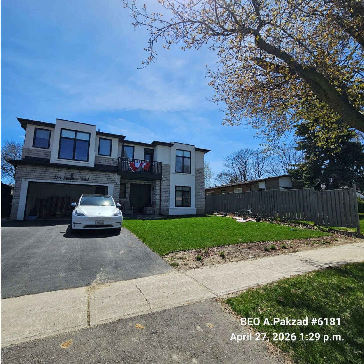
Attachment 2: Supervisor's photo - Overview of fence at 124 Pegasus Trail
