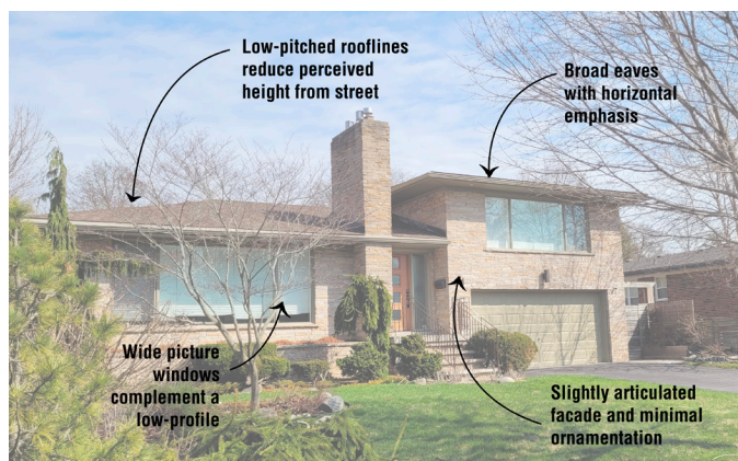
Simple front facade featuring a balance between large horizontal windows and restrained detail.
