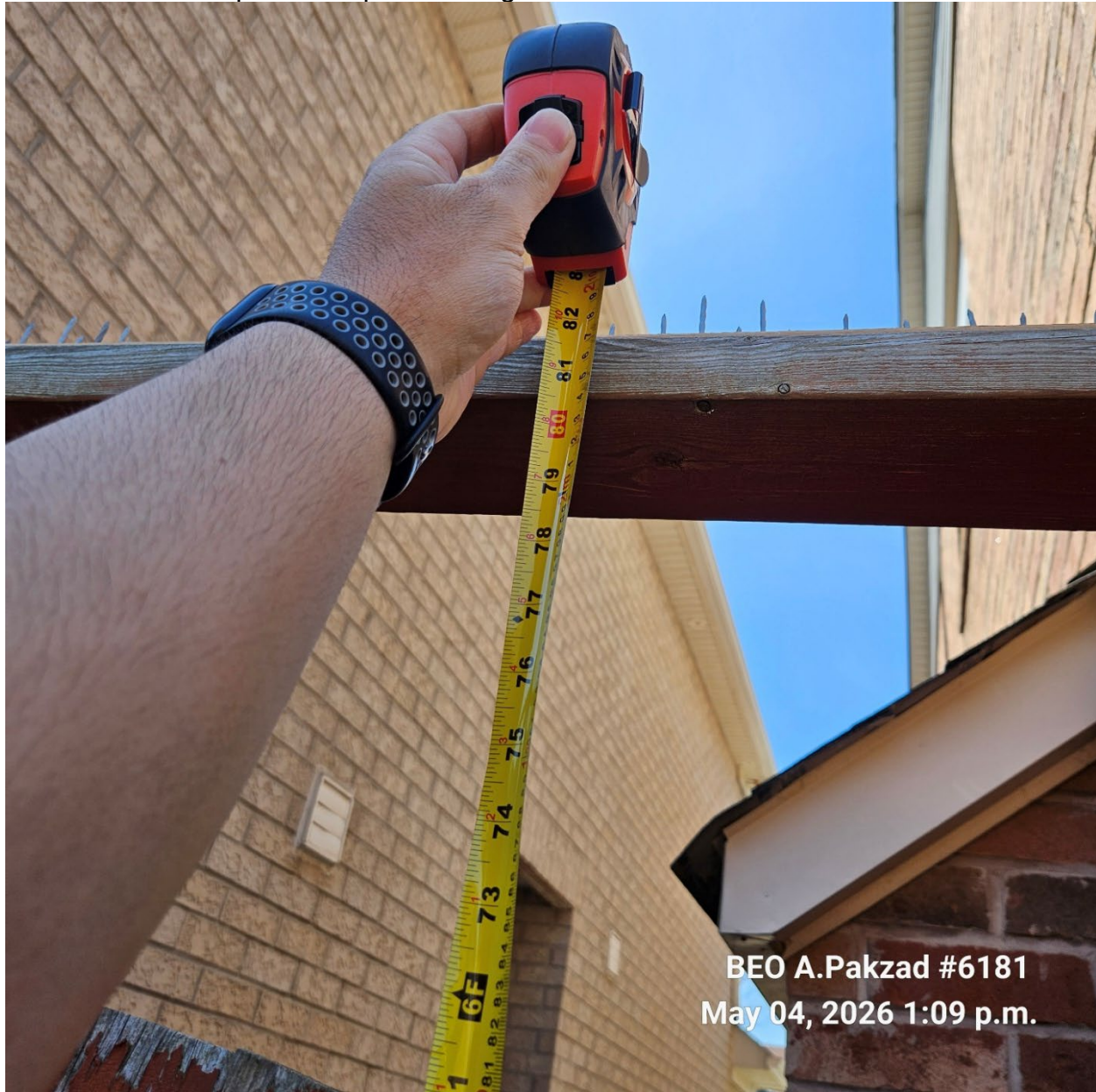
Attachment 10: Supervisor's photo - Height of East Side Gate 2.08m
