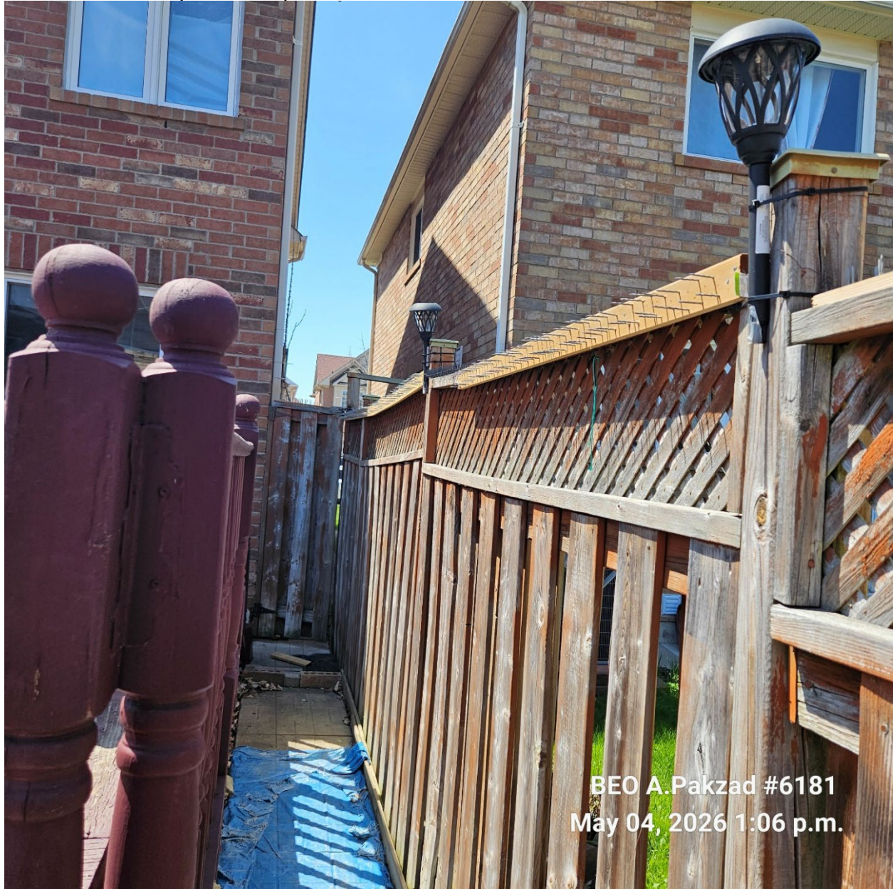
Attachment 3: Supervisor's photo - Overview of Rear Yard West Side Fence
