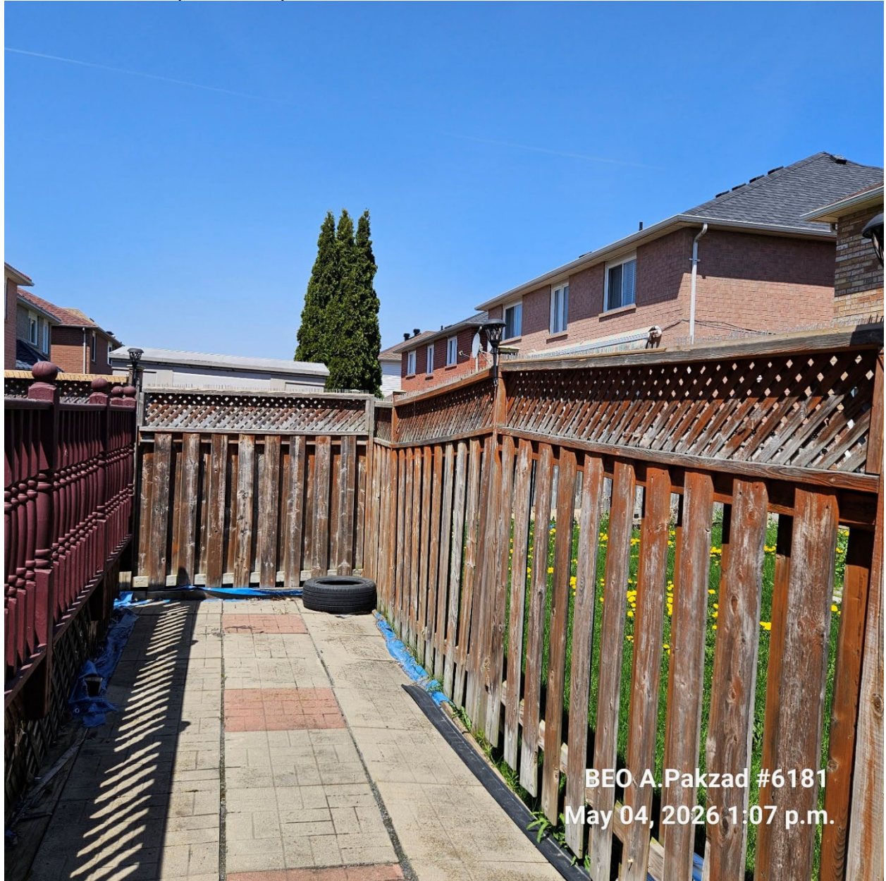
Attachment 4: Supervisor's photo – Overview of Rear Yard North Side Fence
