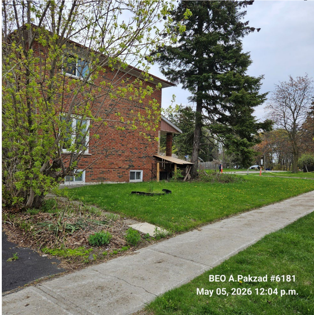
Attachment 3: Supervisor's photo – Overview of Front Yard North Facing
