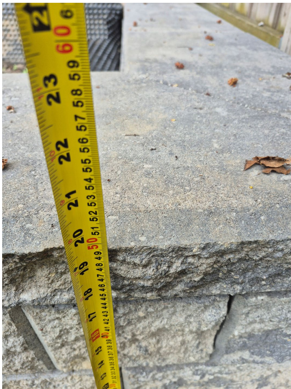
Attachment 3: Supervisor's photo - Retaining Wall/Garden Height (0.5 meters)
