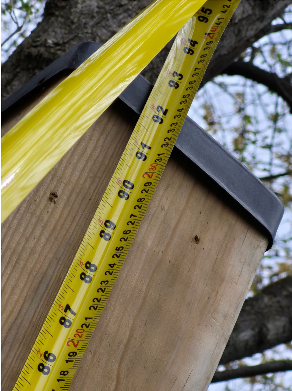
Attachment 4: Supervisor's photo - Rear yard fence- east side - fence height (2.84 meters to 2.87 meters)
