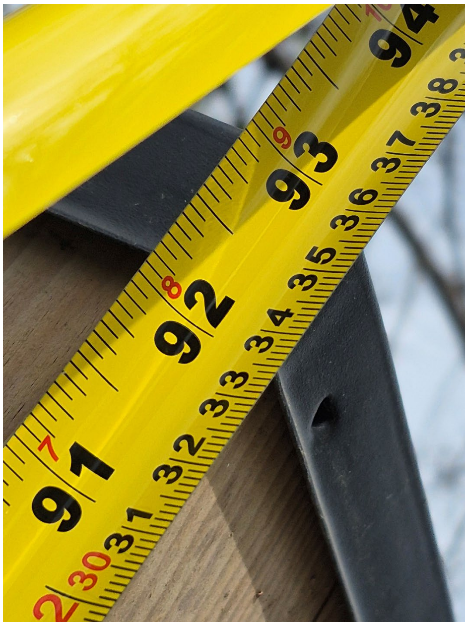
Attachment 6: Supervisor's photo - Rear yard fence- north side - fence height (2.26 meters to 2.87 meters)
