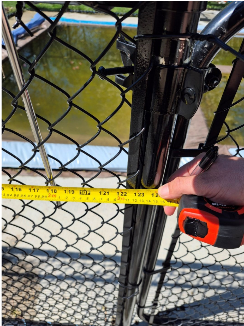
Attachment 4: Supervisor's photo – Pool Enclosure Fence Post Spacing (3.12 meters)
