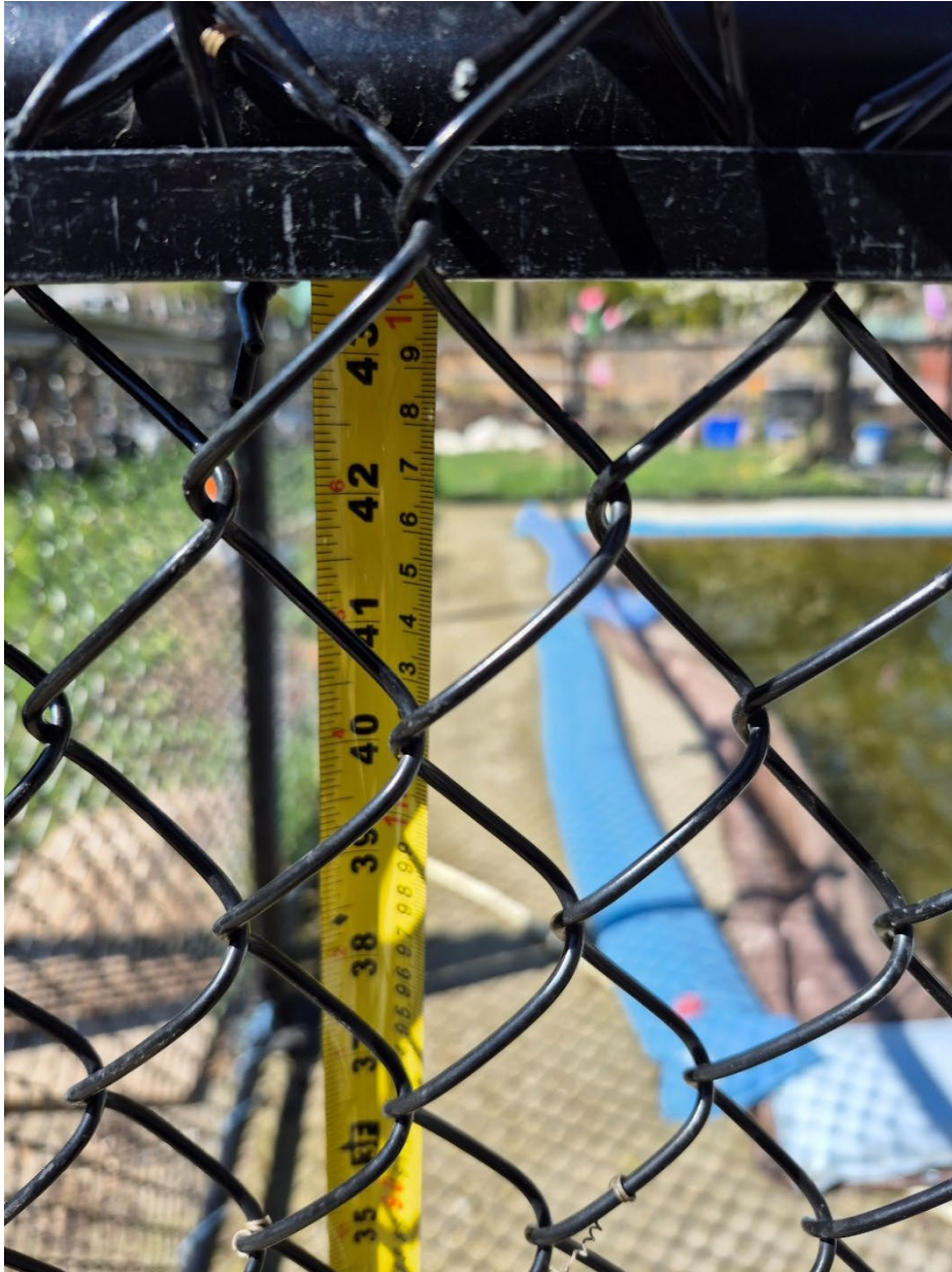
Attachment 3: Supervisor's photo – Pool Enclosure Fence Height (1.10 meters)
