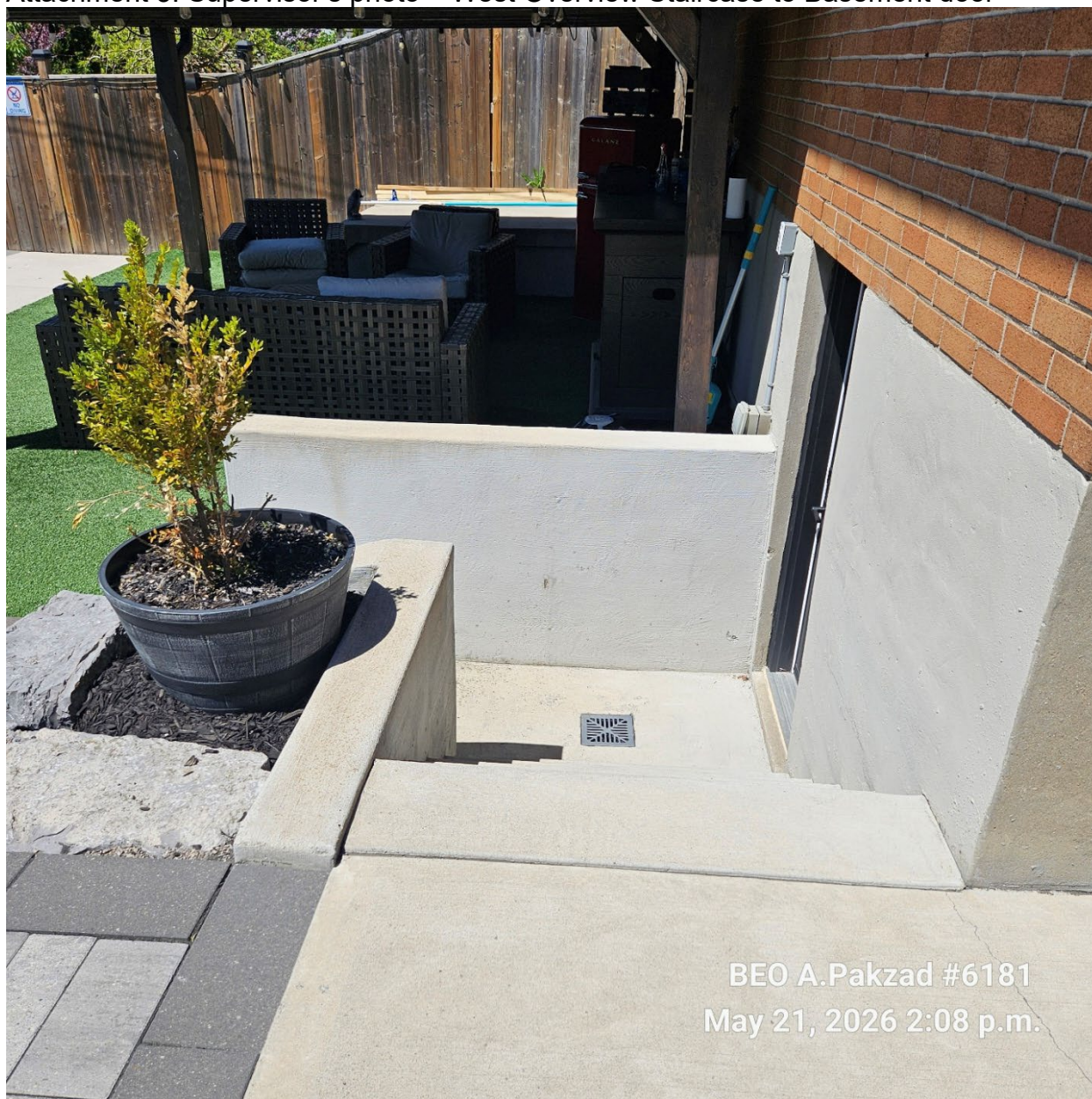
Attachment 3: Supervisor's photo – West Overview Staircase to Basement door
