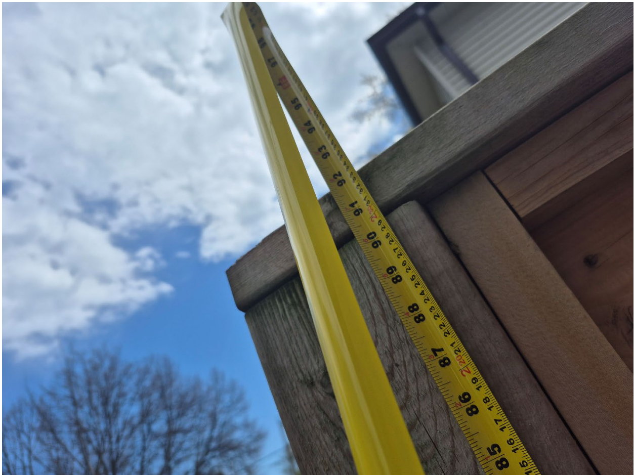
Attachment 12: Supervisor's photo - Front yard fence- south side - fence height (2.34 meters)
