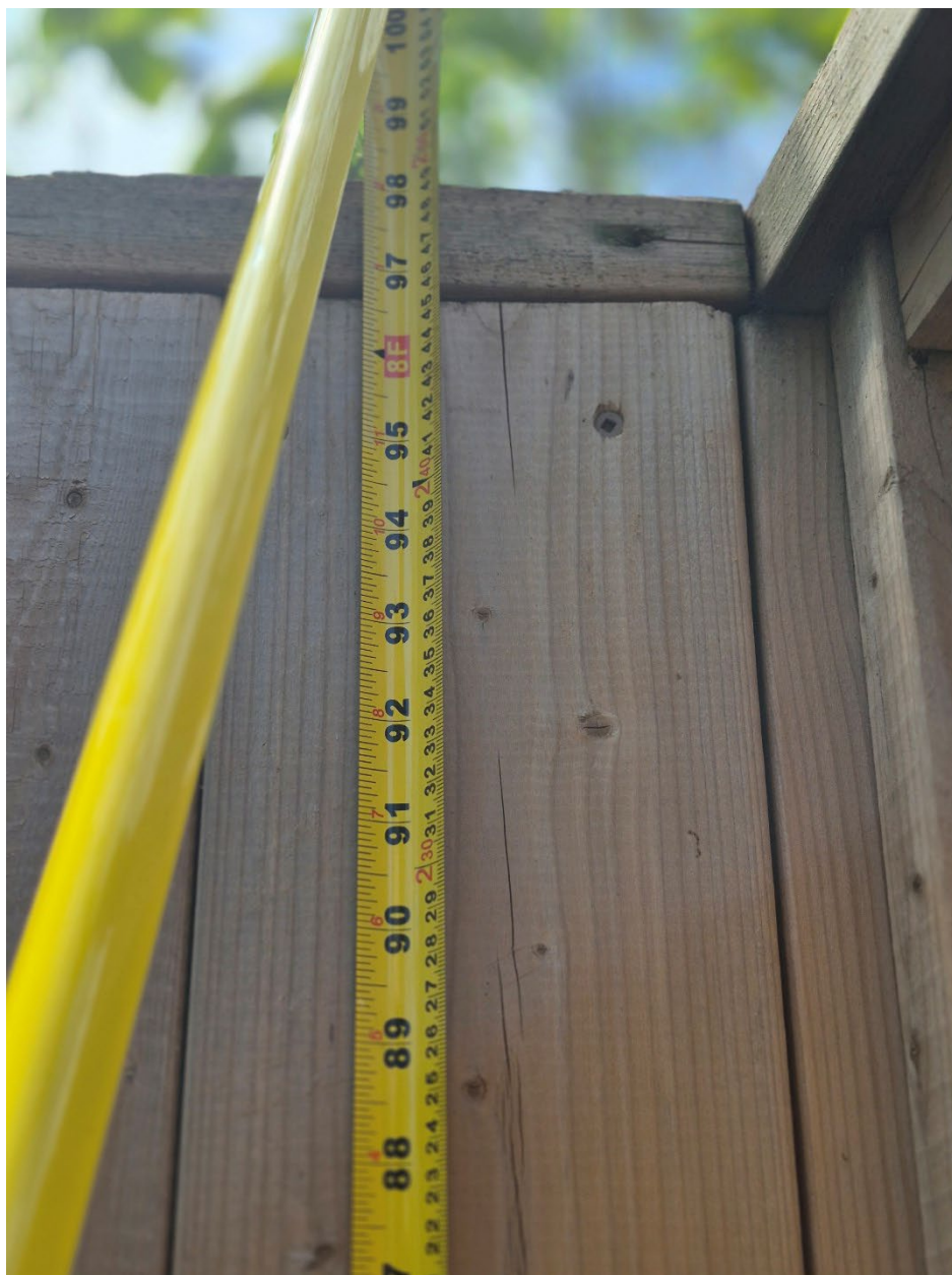
Attachment 5: Supervisor's photo - Side and Rear yard fence- north side - fence height (2.39 meters to 2.49 meters)
