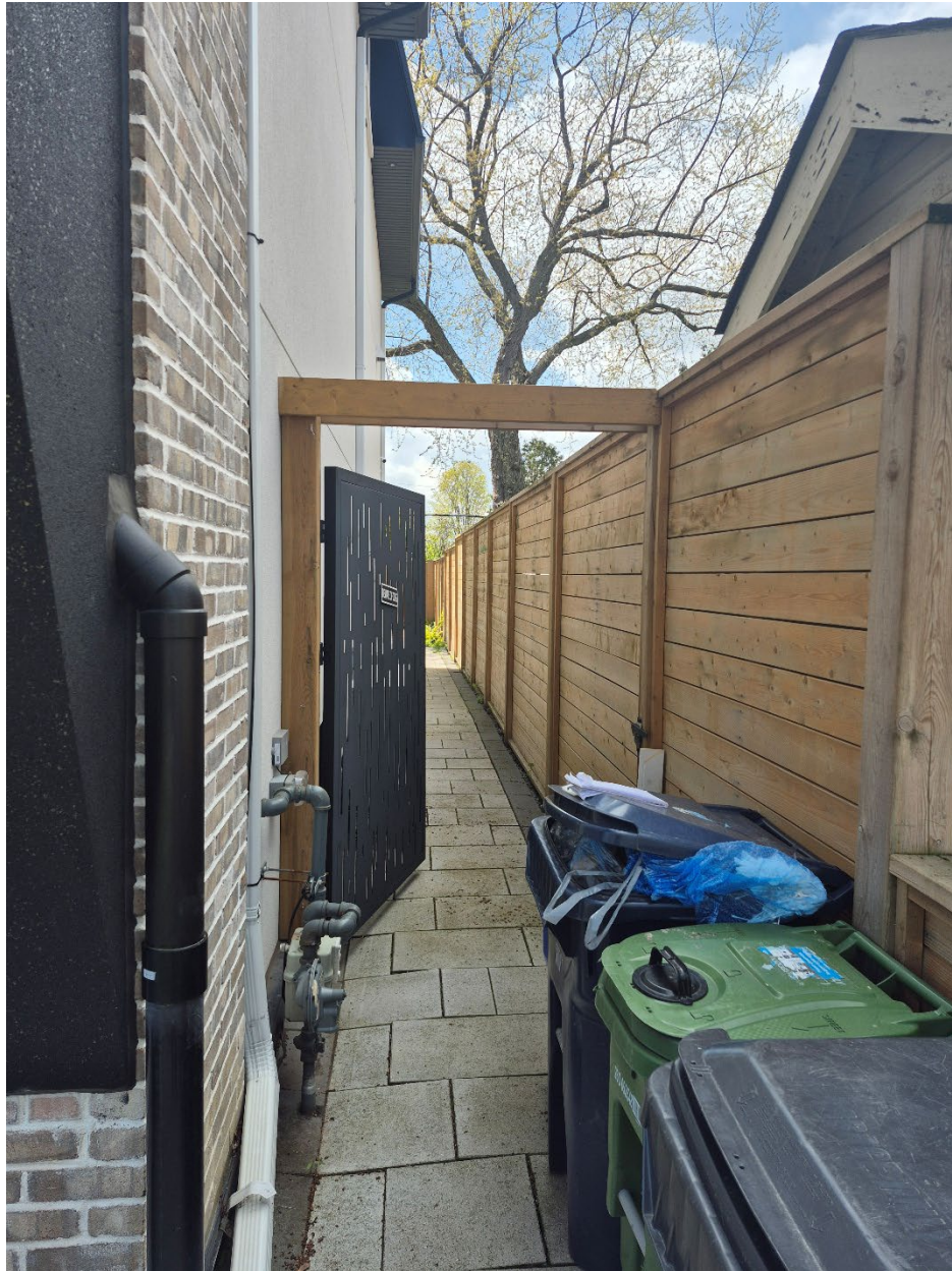
Attachment 3: Supervisor's photo -Overview of Side/rear yard fence/gate- north side.
