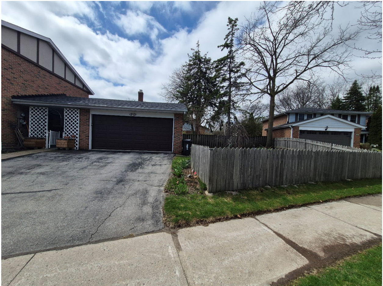
Attachment 7: Supervisor's photo -Overview of rear yard - southeast side (of rear yard)- proposed fence location
