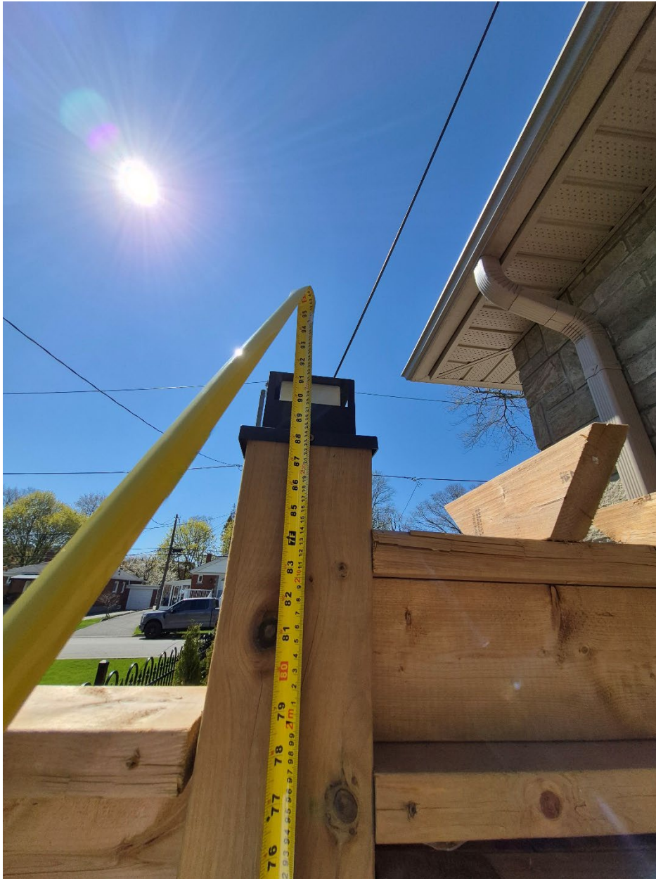
Attachment 9: Supervisor's photo - Side yard gate- east side - gate height (2.32 meters)
