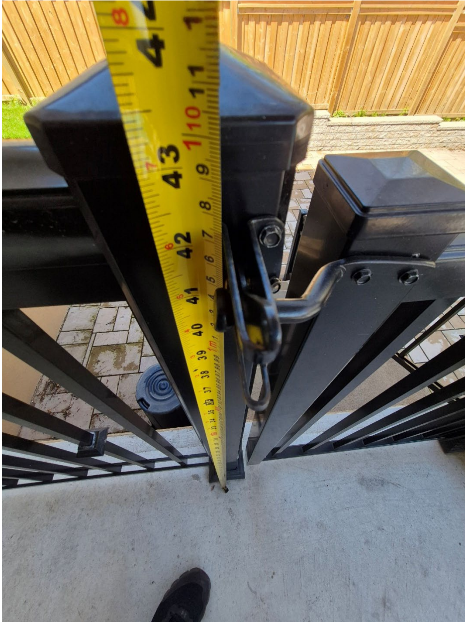
Attachment 15: Supervisor's photo - Gate latch in rear yard- northwest side of house - raised patio/deck- Fence height (1.06 meters)
