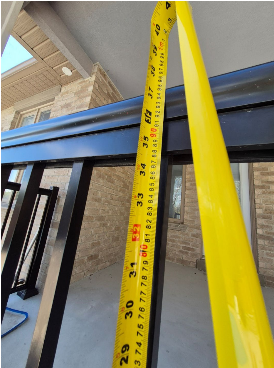
Attachment 14: Supervisor's photo - Fence in rear yard- northwest side of house - raised patio/deck- Fence height (0.94 meters)
