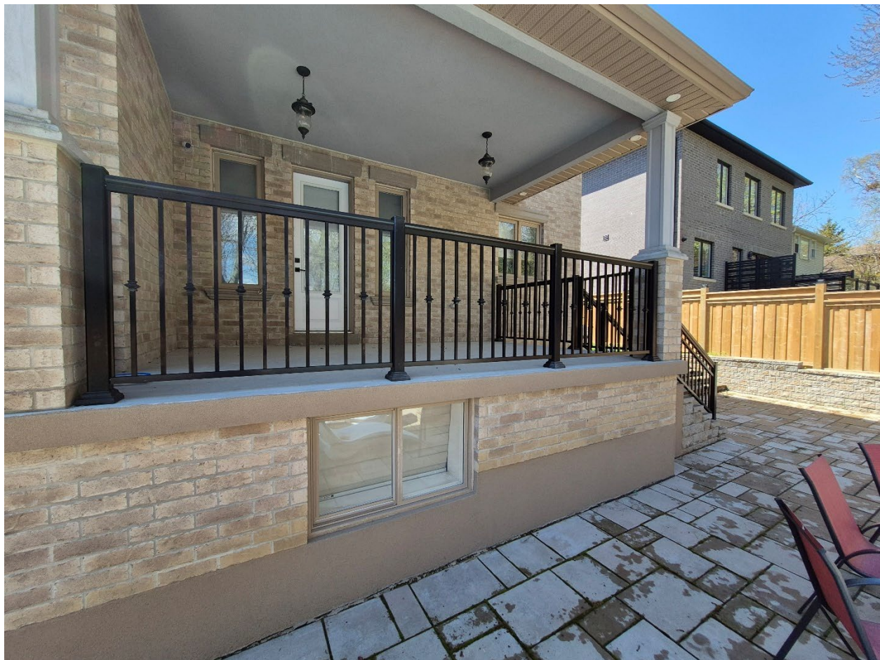
Attachment 13: Supervisor's photo - Overview of fence in rear yard- northwest side of house - raised patio/deck
