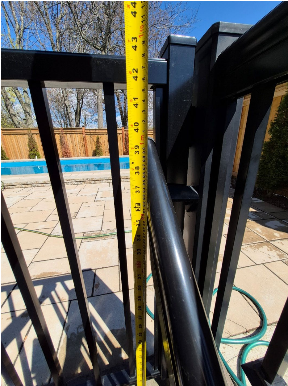
Attachment 12: Supervisor's photo - Fence in rear yard- northeast side of house - stairs to basement- climbable object (less than 1 meter from fence)
