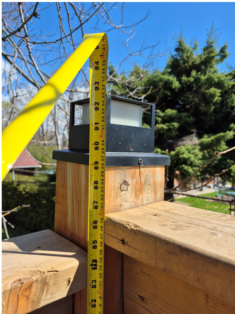
Attachment 8: Supervisor's photo - Rear/side yard fence- east side - fence height (2.32 meters to 2.35 meters)
