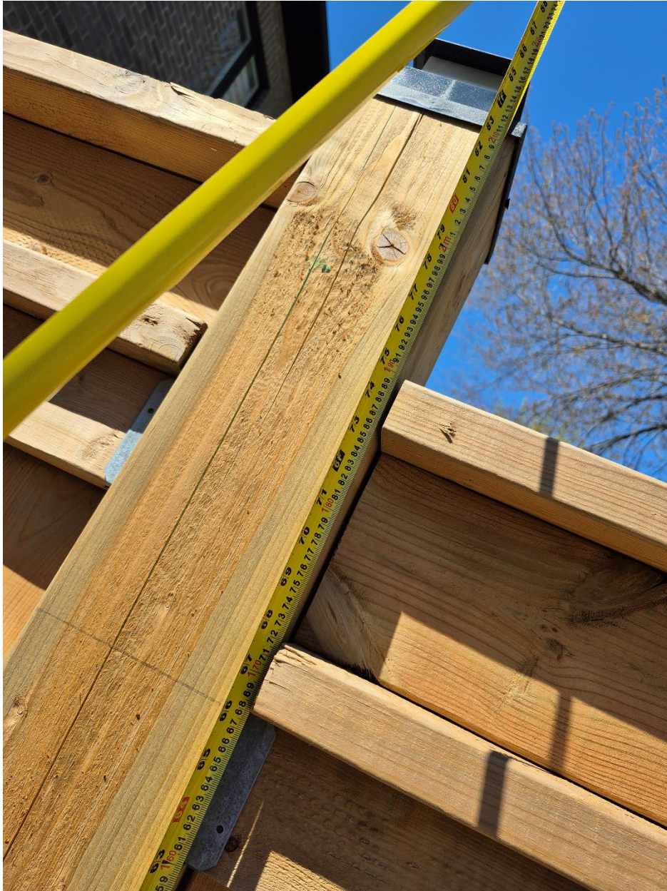
Attachment 5: Supervisor's photo - Rear yard fence- west side - fence height (2.18 meters)
