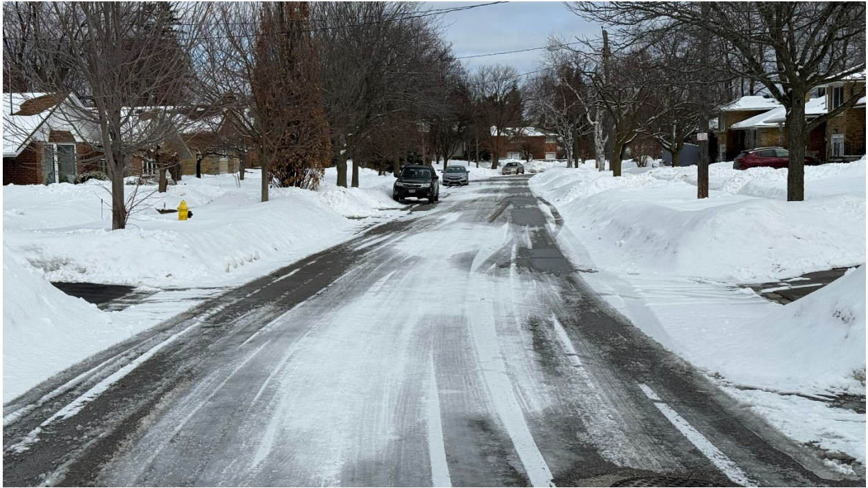
Fig. 6 - Again, due to the challenging road grade changes on Perivale Cres, heavy compacted ice build-up, especially in the centre lane is a very common occurrence. Note, these conditions exist without surface-grade road obstacles like speed humps. (Feb 2026)
