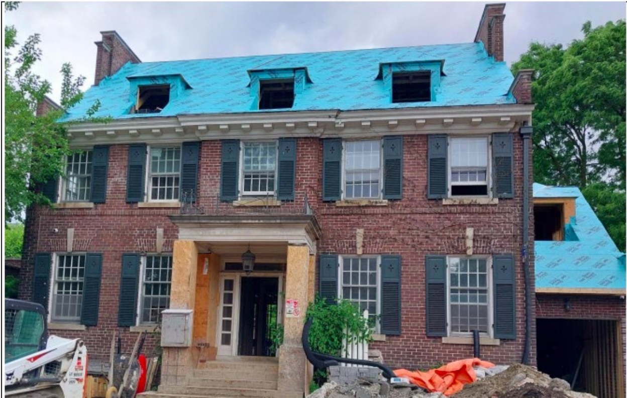
Photograph showing the existing condition of the dwelling (Clifford Restoration Limited).
