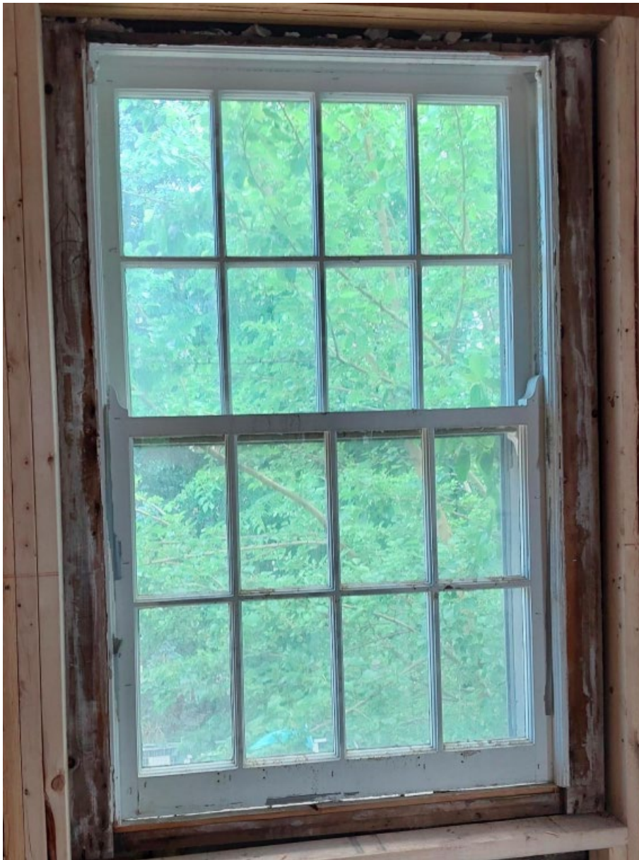
Detail photograph of typical window.
