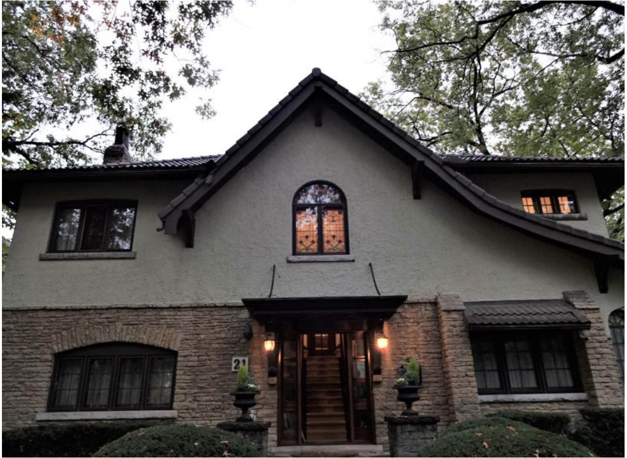
Detailed photo of the front, north elevation of the existing building at 21 Baby Point Crescent prior to the removal of the preexisting door and entrance portico (Starkey Group Architects Inc., 2024).
