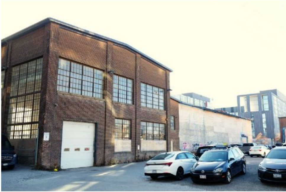
Figure 10: North elevation of 185 Eastern Avenue (Machine Shop building), looking south (Philip Goldsmith Architect, 2025).
