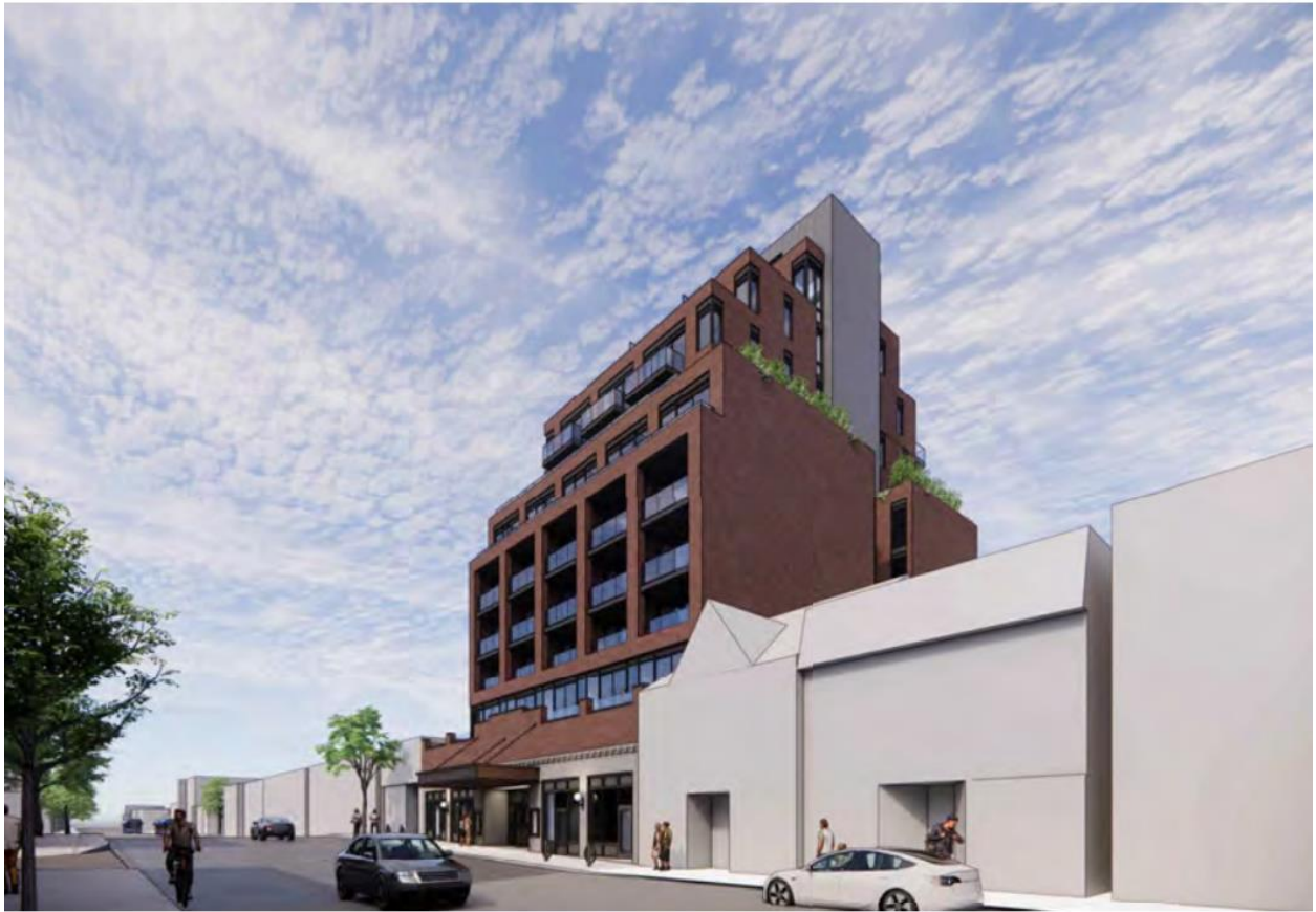
Figure 15. Proposed primary (west) elevation of 509 Parliament Street, rendering looking northeast (ERA Architects Inc., 2025).
