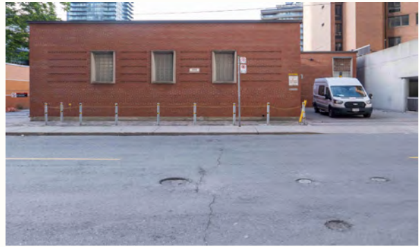
TTC Substation building at 30 Asquith Ave. (CBCollective 2021).
