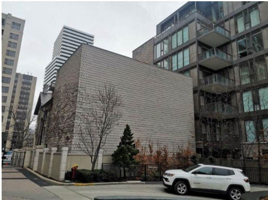
North elevation of 8 Prince Arthur Avenue showing the three storey concrete block rear addition. The proposed new addition will be built on top of this portion of the existing building (Source: GBCA Architects, 2026)
