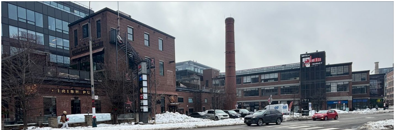
On the left is the building at 165-167 East Liberty Street (north elevation) and on the right is the building at 171 East Liberty Street (east elevations) (City of Toronto Heritage Planning, 2026)
