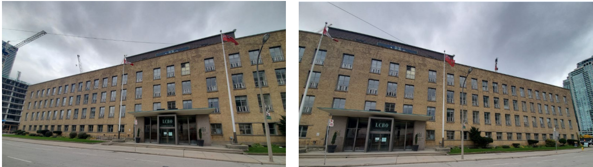
Figure 2a and 2b: Details of the principal (north) elevation of the LCBO Office Building (Heritage Planning, 2020)
