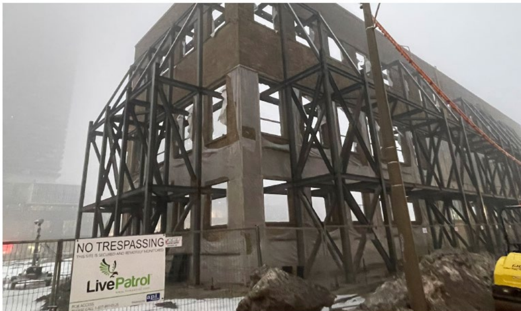
Figure 11: North and west elevation of the Warehouse Building, looking southeast (Giaino + Associates Architects Inc., 2026).
