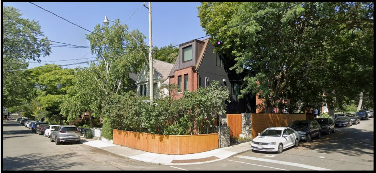
Looking northwest at 16 Afton Avenue
