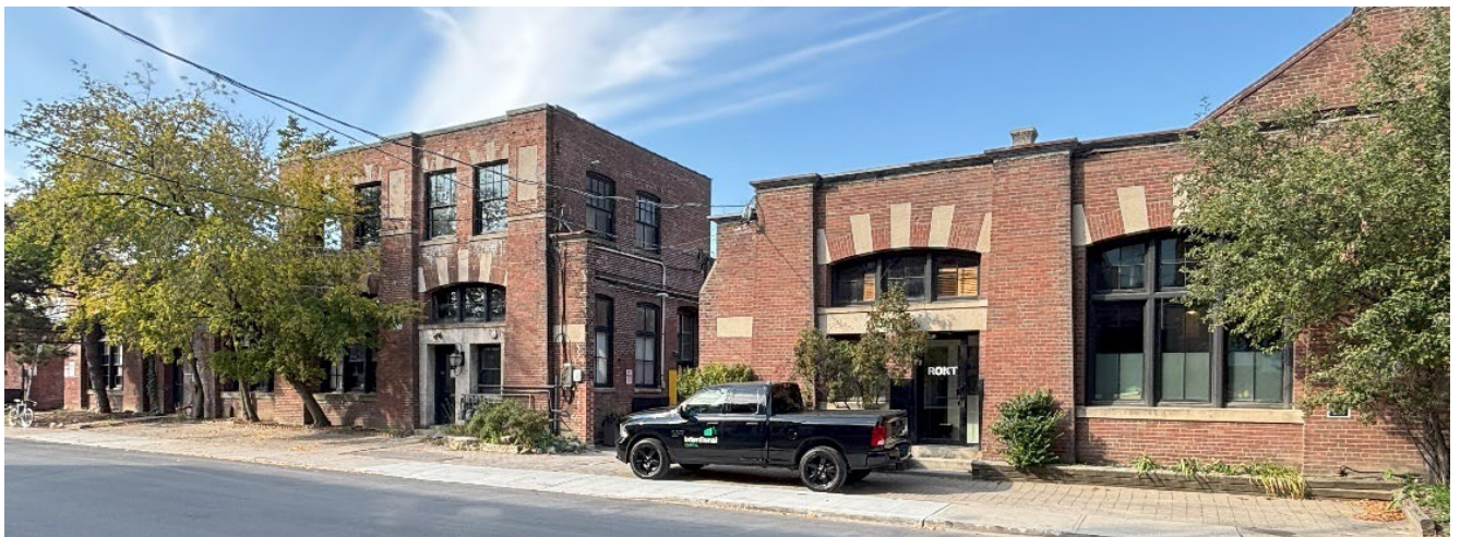
54-66 Fraser Avenue: East/Street Facades
