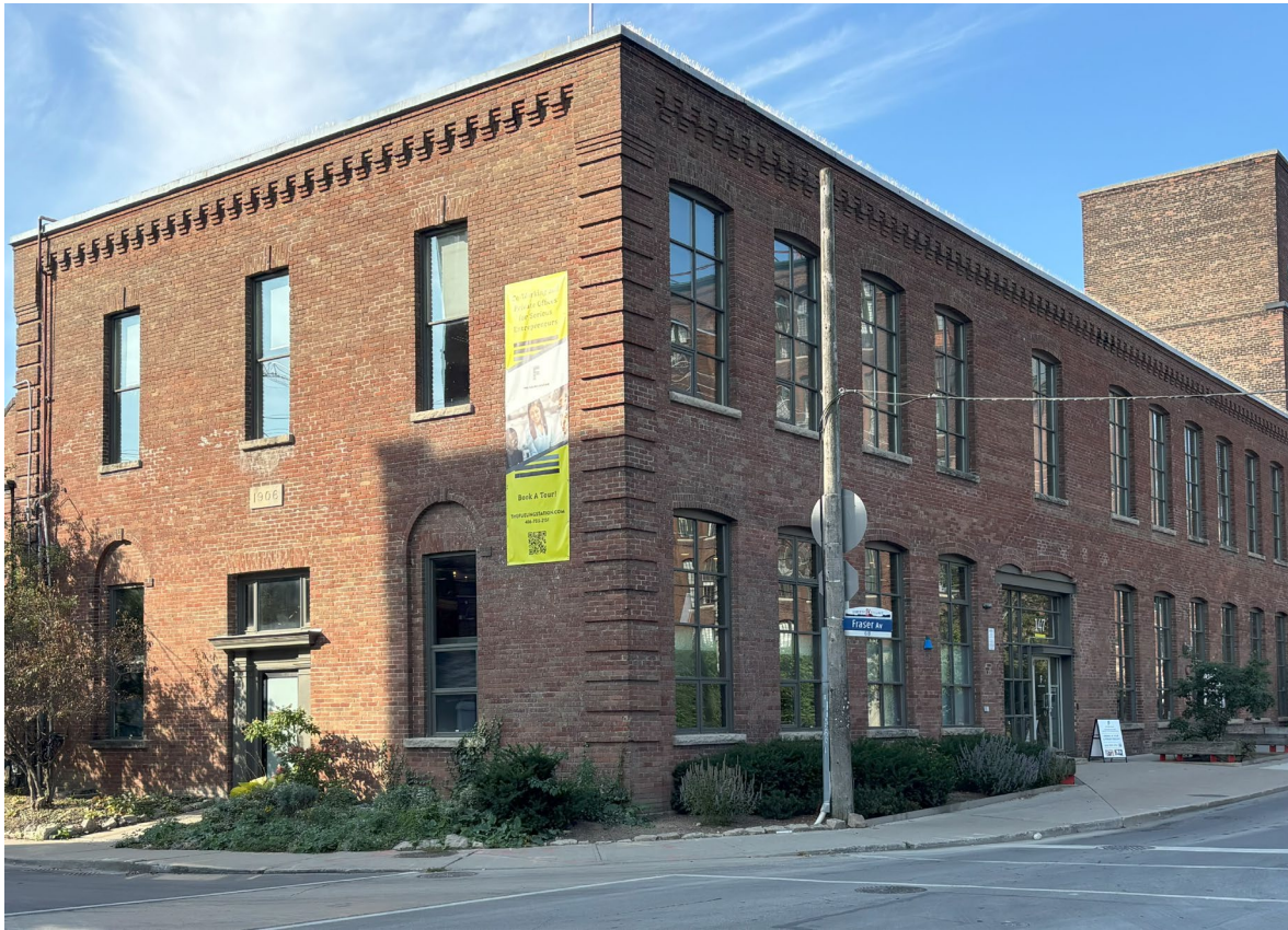
68 Fraser Avenue (147 Liberty Street): East and North Facades at Northeast Corner at Fraser Avenue and Liberty Street
