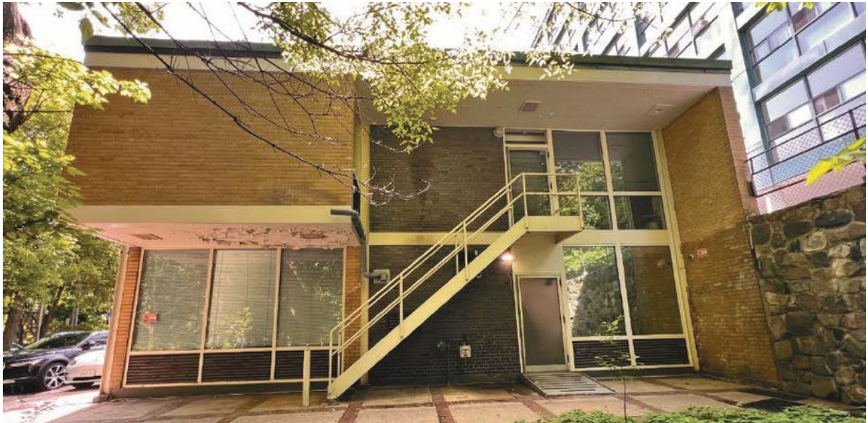
West elevation of 50 Park Road (ERA Architects, 2025)
