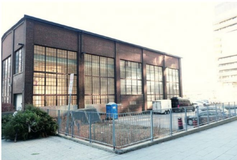
Figure 9: East elevation of 185 Eastern Avenue (Machine Shop building), looking west (Philip Goldsmith Architect, 2025).
