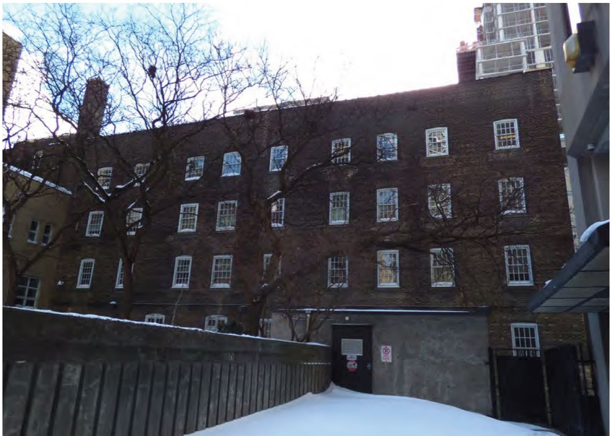
Figure 5: Rear (north) elevation of 20 Gerrard Street East (ERA Architects Inc., 2026).
