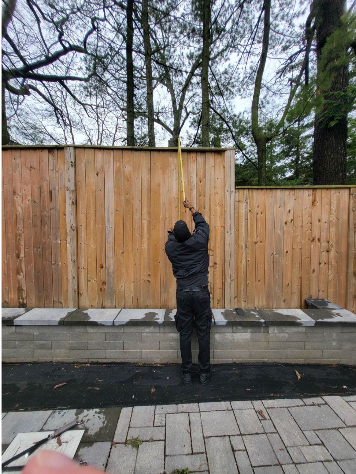
Attachment 12: Rear fence – Western lot line at stone planter
