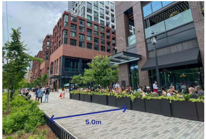
Figure 40. The wide sidewalk at La Plume in The Well supports the pedestrian experience and enhances walkability
