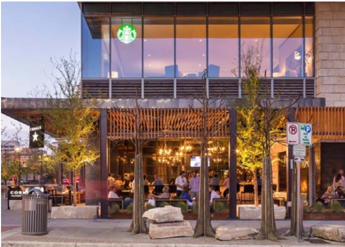
Figure 18. Building design creates a strong relationship to public realm (Austin, Texas)
