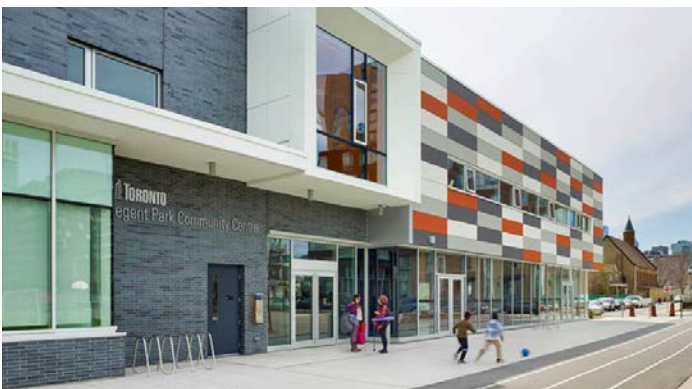
Figure 36. Frequent ground level entrances, variation in colours, materials and building articulation contribute to an attractive and active facade along the length of the building (Regent Park Community Centre)
