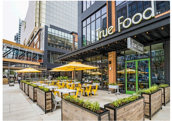
Figure 29. Signage integrated to complement architectural form (Arlington, Virginia)
