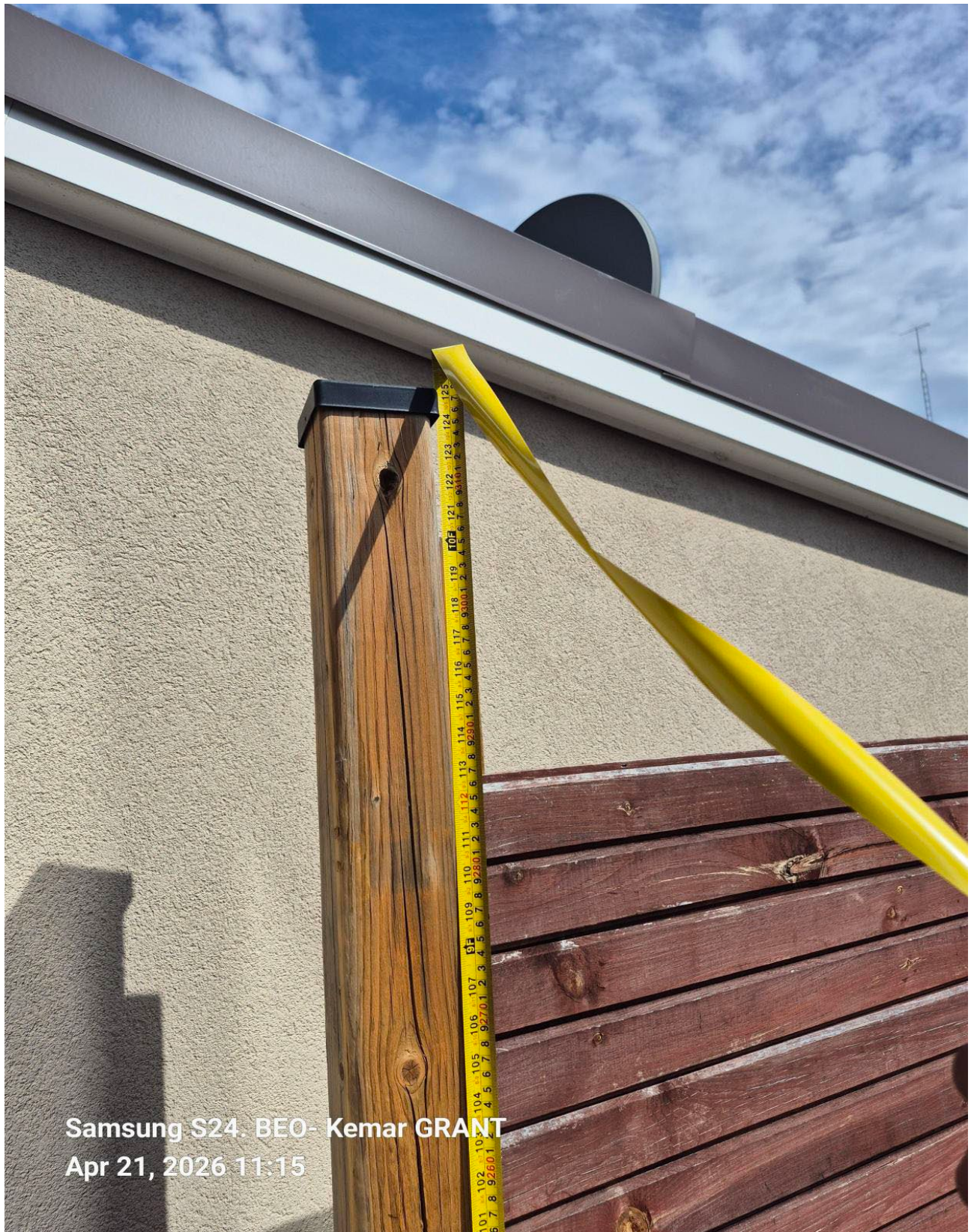
Attachment 4: Rear fence post – Northern lot line first panel post from rear deck
