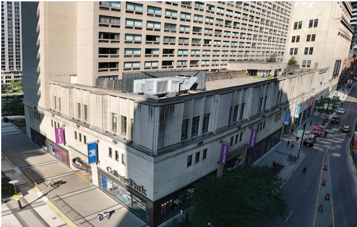
College Park, Looking northwest at South Façade and Yonge Street/East Façade
