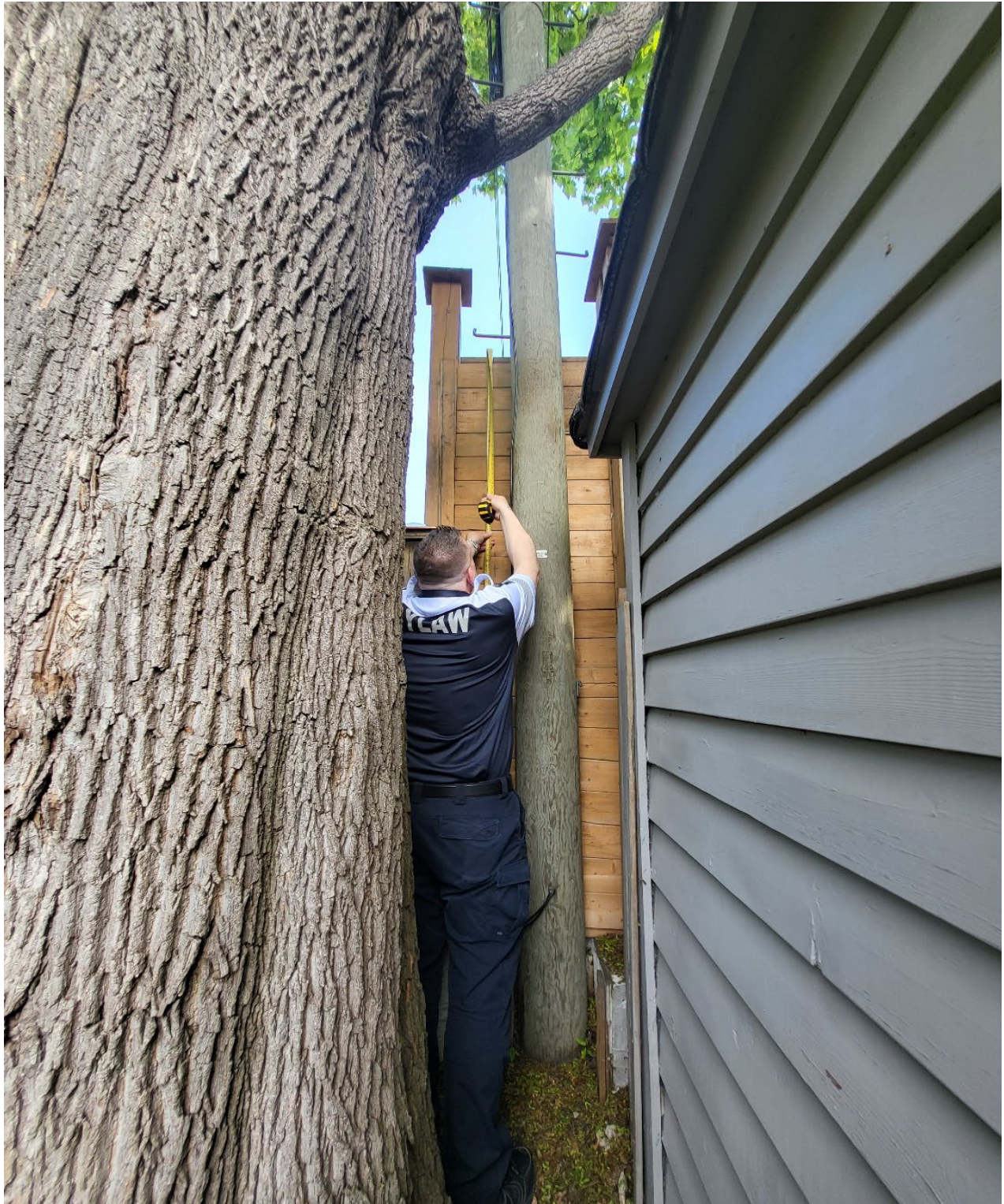
Attachment 11: Rear fence – West lot line from 59 High Park Boulevard's grade
